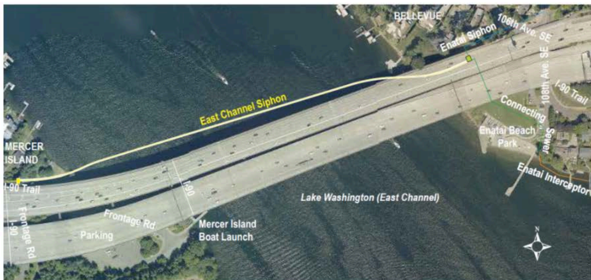
East Channel Crossing Overview
