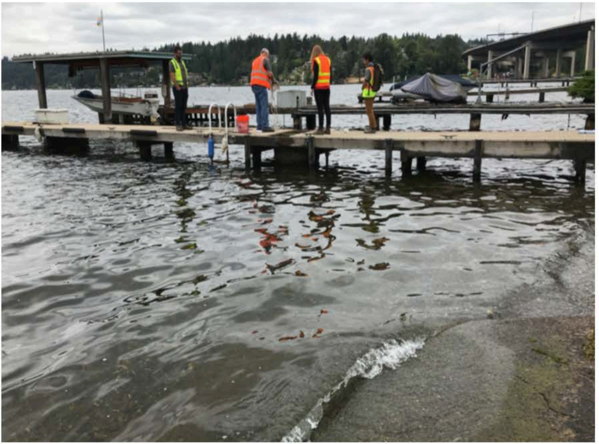
The existing pipeline will be accessed from the various maintenance holes that run along the line from Enatai Beach Park, under some docks, and up the Mercer Slough.
