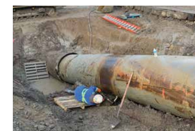
Preparing the site at Sveyolocken for the HDD pipe pull.
