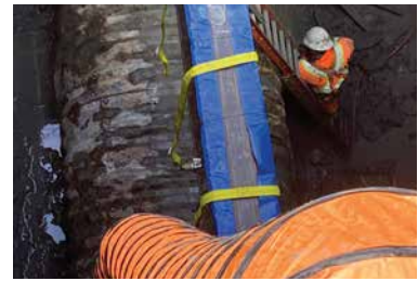
Air vents circulate fresh air for crew members working underground.
