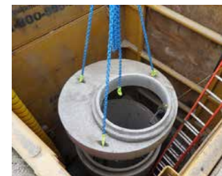
Crews install a maintenance hole where two pipes connect.
