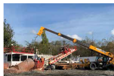
Crew members install a flange plate, which allows pipe segments to be easily screwed together.
