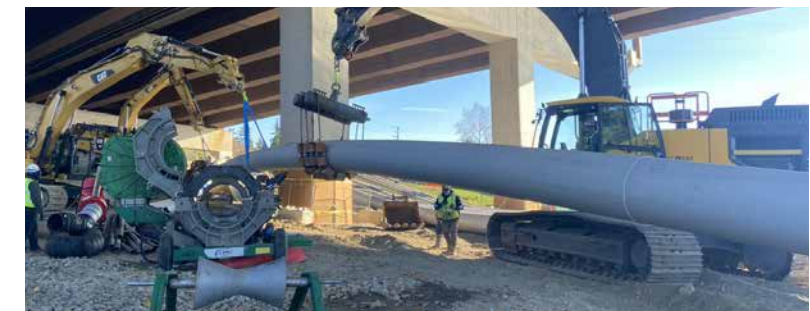
Feeding the pipe into the HDD hole by Enatai Beach Park.
