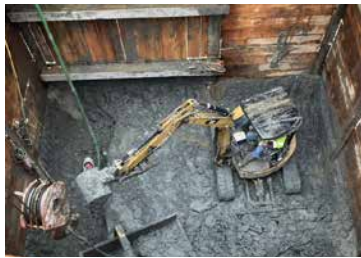
Excavators dig the base for the temporary pump station.
