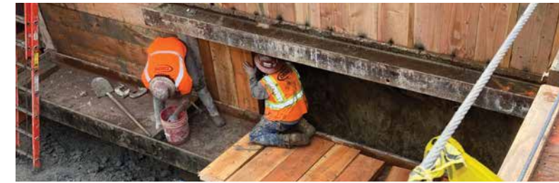
Crews build a retaining wall and install wooden panels, called lagging, to hold back the ground before building the temporary pump station.
