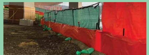
A silt fence protects waterways from debris at the construction staging area.
