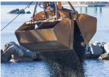
Dredging is the first step for in-water pipe installation.
