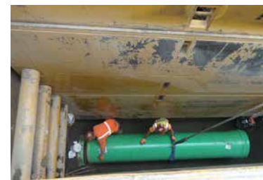
Shoring holds back the soil so that crews can safely work below the surface grade.
