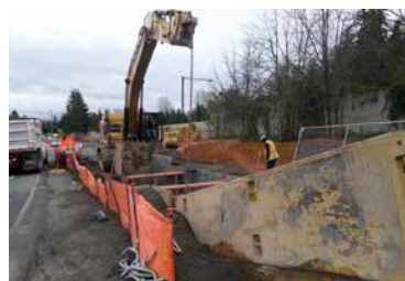
Shoring boxes allow crews to safely work below the ground.
