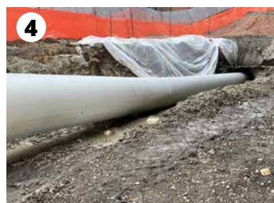
Photos: 1: 3,000 feet of fused pipe were floated on Lake Washington before the pipe was pulled under the Enatai hillside. 2: A crane lifted the new sewer pipe out of the water in preparation for underground installation. 3: Feeding the pipe into the HDD hole by Enatai Beach Park. 4: A rig at Sweyolocken pulls the end of the pipe line through the pipe path. 5: The new sewer pipe entered the pipe path at Enatai Beach Park.
