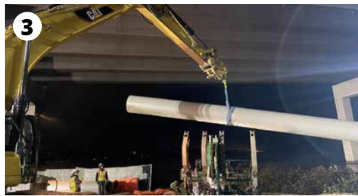
Photos: 1: 3,000 feet of fused pipe were floated on Lake Washington before the pipe was pulled under the Enatai hillside. 2: A crane lifted the new sewer pipe out of the water in preparation for underground installation. 3: Feeding the pipe into the HDD hole by Enatai Beach Park. 4: A rig at Sweyolocken pulls the end of the pipe line through the pipe path. 5: The new sewer pipe entered the pipe path at Enatai Beach Park.
