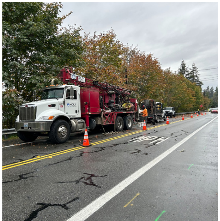
Geotechnical work along East Lake Sammamish Parkway.
