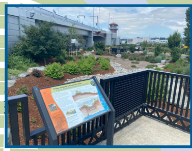
4 SOUTH PARK BRIDGE 14th Ave S and S Orr St
