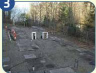
Sewage is treated using a series of sand filters and septic tanks. Pollutants settle out in the tanks. Solid material is consumed by good bacteria in a sand filter. UV light is used to disinfect treated water.
