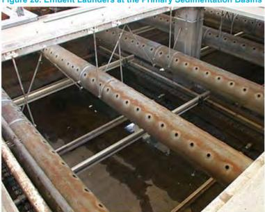
Figure 20. Effluent Launders at the Primary Sedimentation Basins
