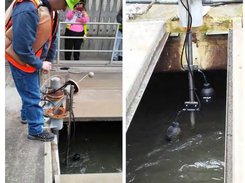
Figure 28. New Float Switches Being Tested and Shown as Installed at West Point Treatment Plant
