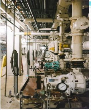
Gravity Belt Thickener Feed Pumps - Ready for replacement motors
