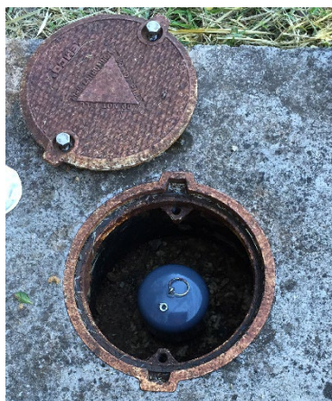
Figure 2. Photograph of a groundwater-monitoring well. Photo taken by Jack Mitchell, February 2, 2018.
