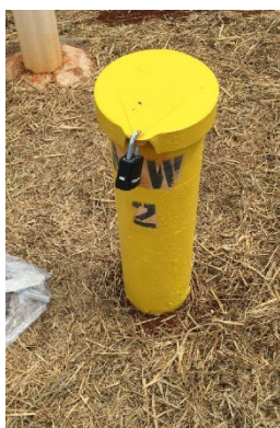
Figure 4. Photograph of a groundwater-monitoring well. Photo taken by Jack Mitchell, January 29, 2018.
