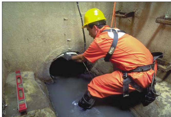
Figure C2 Installation of Open Channel Area-Velocity Metering Equipment
