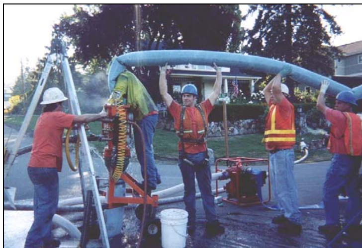
Crew installing cured-in-place-pipe (CIPP) using air inversion method.
