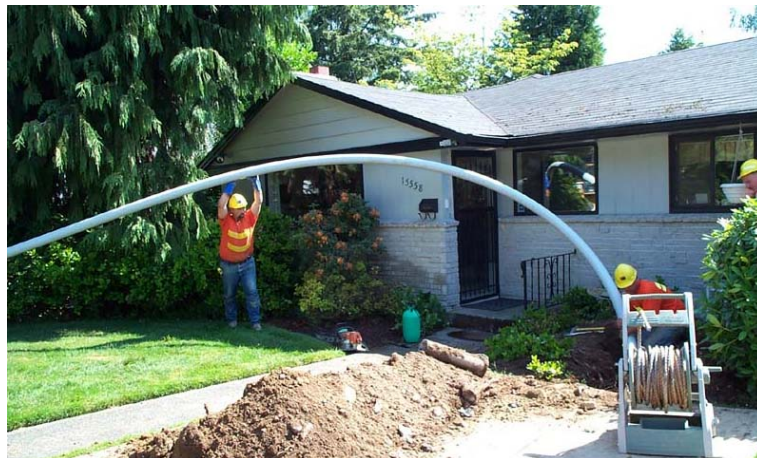
Relining a side sewer on private property.
