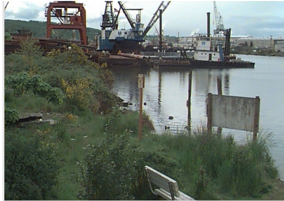
8th Avenue South Regulator Station CSO Vicinity; Looking Northwest Across Duwamish River
