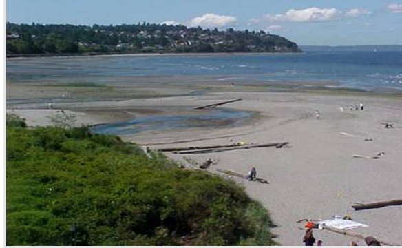
Carkeek Wet Weather Treatment Station Vicinity; Beach Looking Southwest
