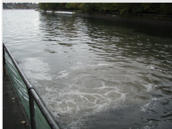
Montlake Regulator Station CSO Overflowing 10/26/09
