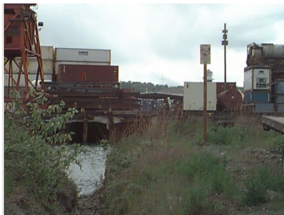
Vicinity of East Marginal Way Pump Station CSO; Looking North Across Slip 4
