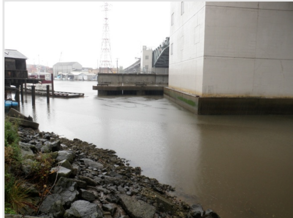
West Michigan Regulator Station CSO Overflowing 10/17/2009
