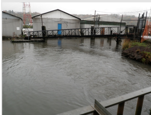
South Michigan Street Regulator Station CSO Overflowing 10/26/09
