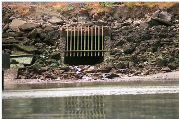
Harbor Avenue Regulator Station CSO/Seattle Storm Drain Outfall at Extreme Low Tide
