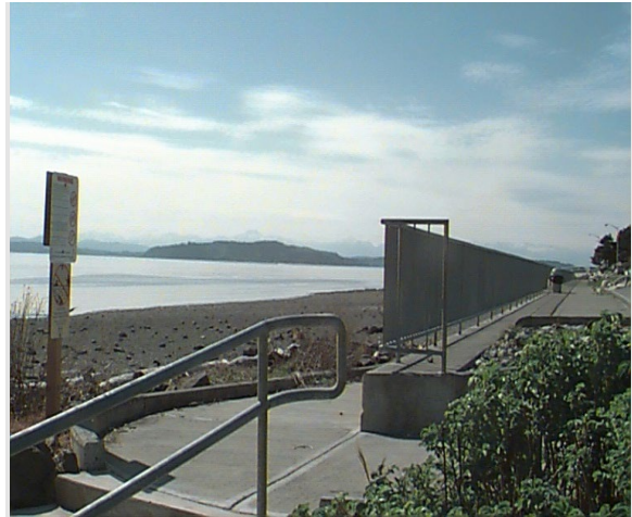
63rd Avenue Pump Station CSO Vicinity; Looking Northwest Across Puget Sound.
