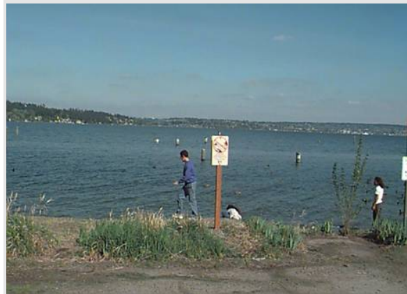
Matthews Park Pump Station CSO Vicinity; Looking Southeast
