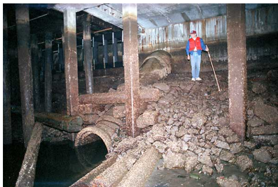
King Street Regulator CSO Outfall at Extreme Low Tide
