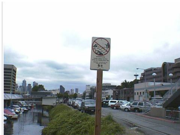
Dexter Avenue Regulator Station CSO Vicinity, Looking South, Parallel to Westlake Avenue
