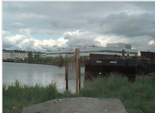
8th Avenue South Regulator Station CSO Vicinity; Looking East Along Duwamish River
