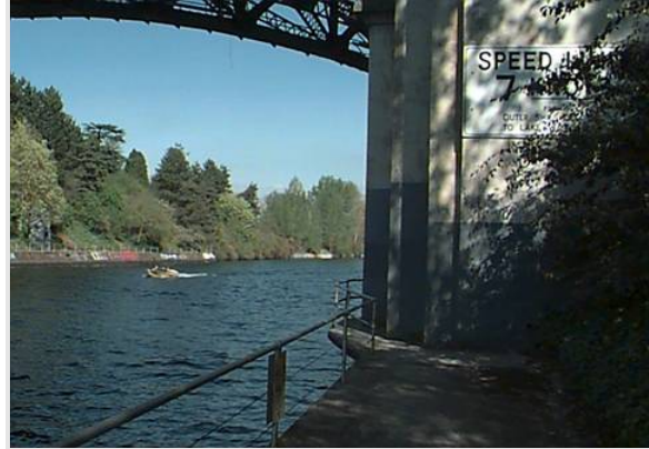
Montlake Regulator Station CSO Vicinity Looking East
