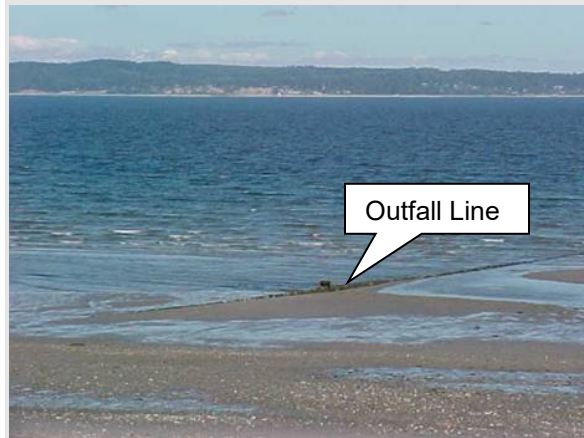
North Beach CSO Wet Well Overflow Outfall; Looking West Across Puget Sound
