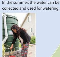
A **cistern** is a large above-ground container used to collect roof water. It is like a huge rain barrel and can hold
