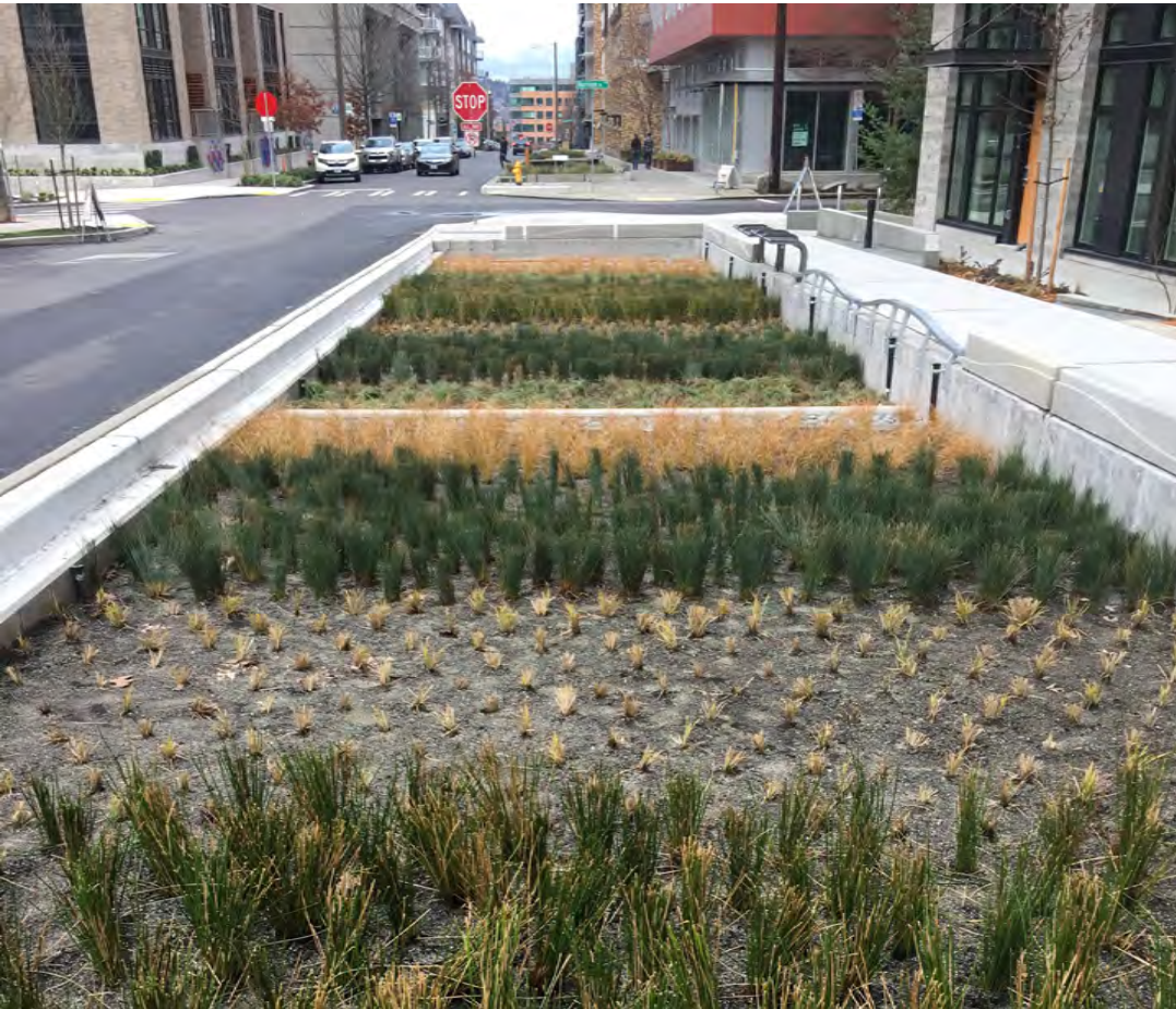
Bioswale on Yale Avenue in South Lake Union.
