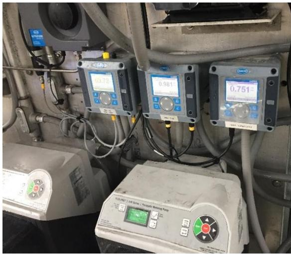
Instrument Displays (pH, TSS, and turbidimeter)
