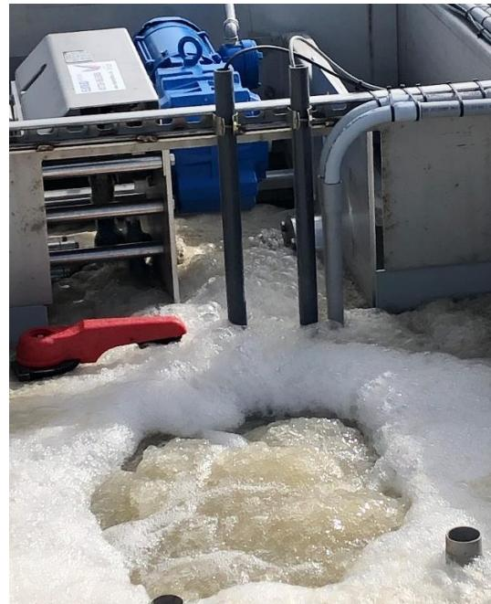
Submerged Screen Box Next to Membrane Tank
