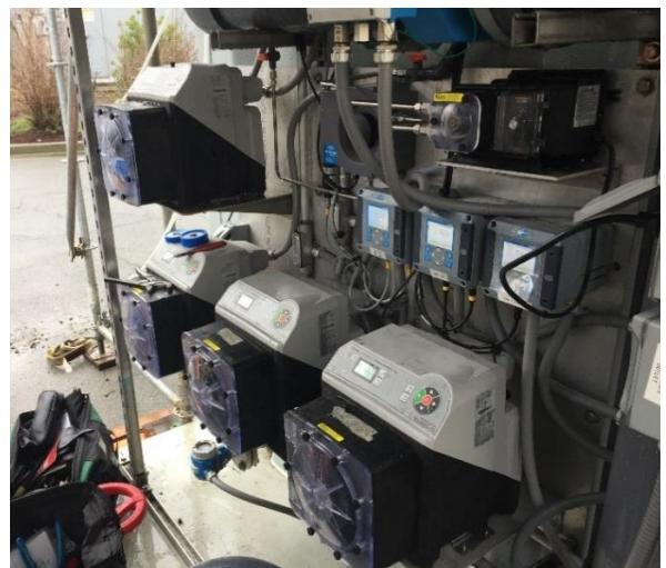
Chemical Feed Pumps and Instruments
