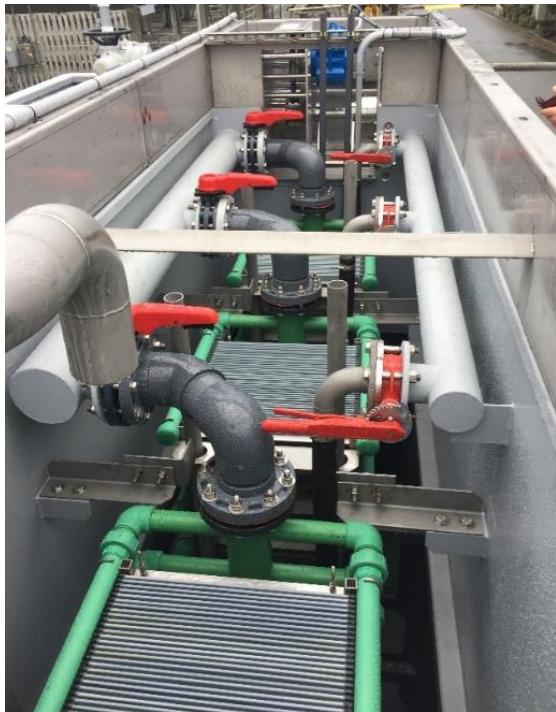
Membrane Tank with Towers – Head Box in Background
