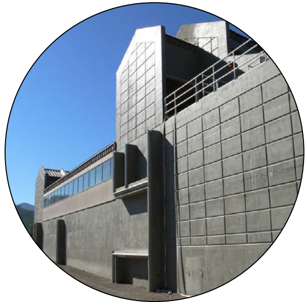
10 MGD Tahoe-Truckee SD BIOSTYR - Truckee, CA
