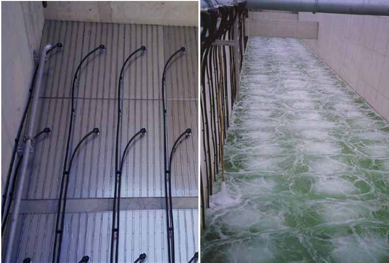
FIGURE 8 – MESSNER PANEL INSTALLED / AERATION PATTERN TEST
