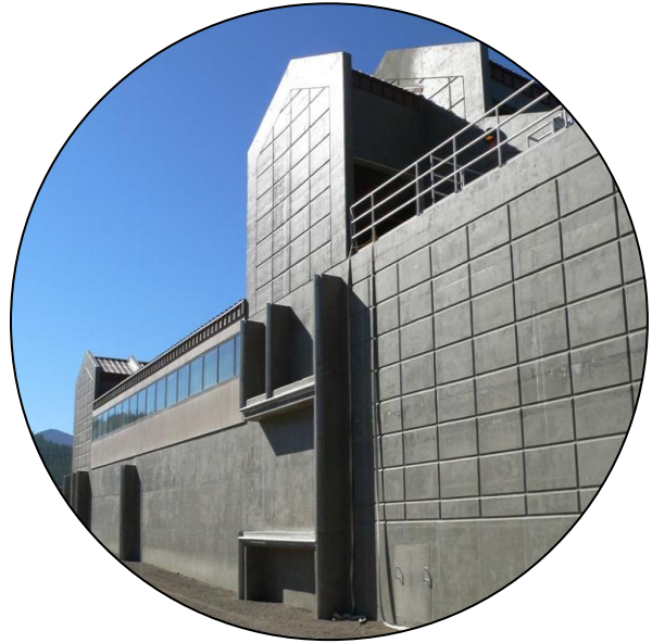
10 MGD Tahoe-Truckee SD BIOSTYR - Truckee, CA
