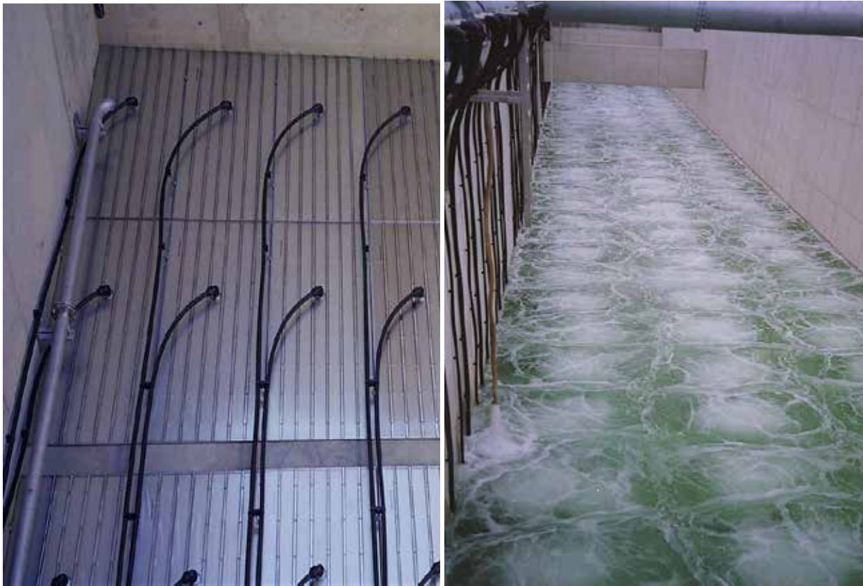
FIGURE 8 – MESSNER PANEL INSTALLED / AERATION PATTERN TEST
