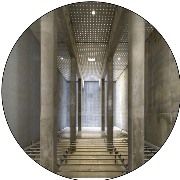
Interior of BIOSTYR Cell
