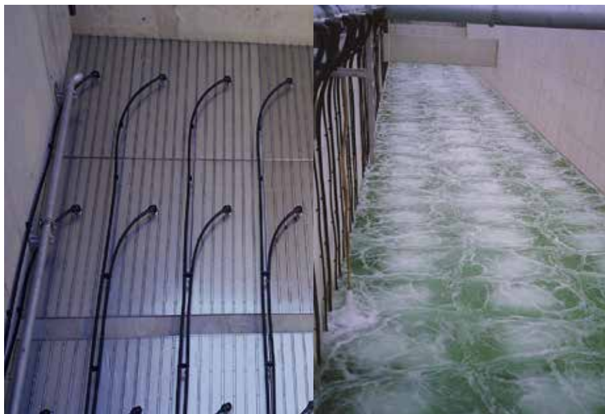
FIGURE 7 – MESSNER PANEL INSTALLED / AERATION PATTERN TEST
