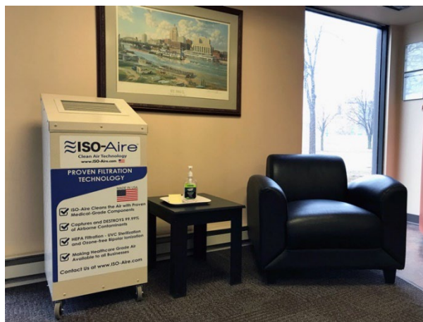
Figure 14. Commercial HEPA air cleaner located in reception lobby to improve IAQ.
