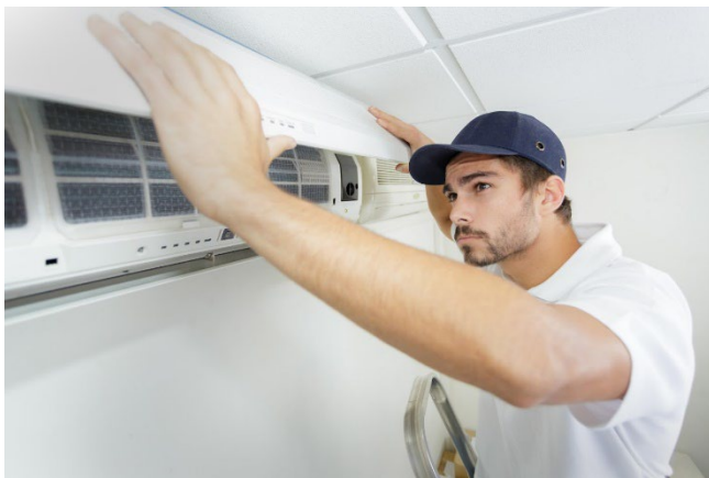
Figure 11. HVAC technician completes installation of ductless heat pump.
