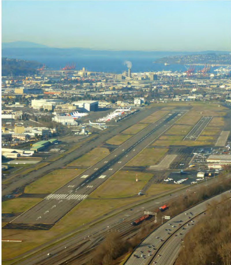
King County International Airport showing Runway 14R-32L and Taxiway B Credit: King County
