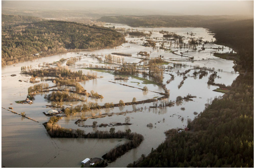
Flooding along the Snoqualmie River in 2015
