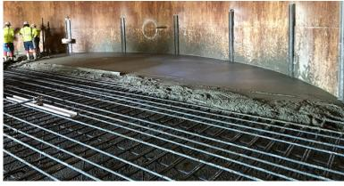
2019: Seismic retrofits at the District's 2 million gallon tank included the pouring of a concrete pad and installing steel stiffeners on the inside walls.
