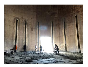
2019: The District installed steel stiffeners inside the 2 MG tank to provide stability during seismic events. Note the size of the workers for scale.
