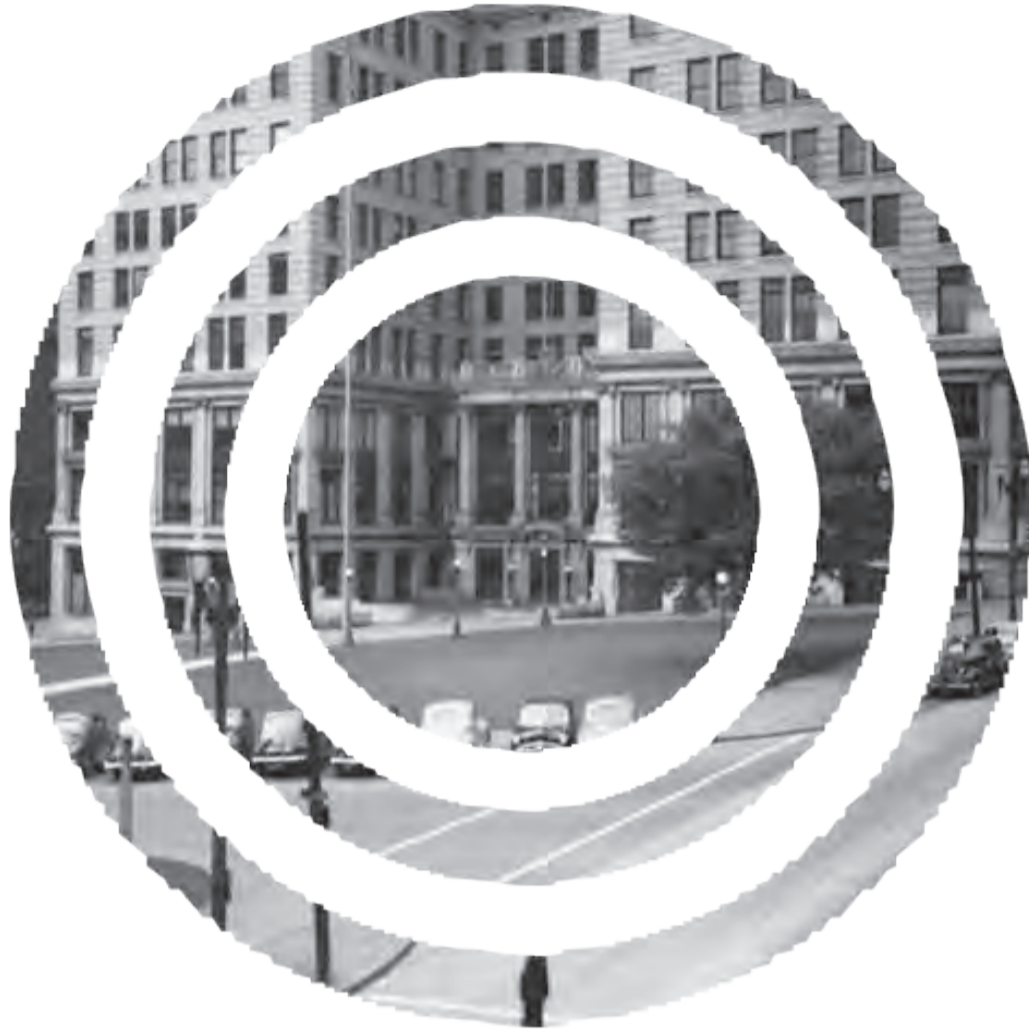
Reclaim the southern entry to the King County Courthouse.
