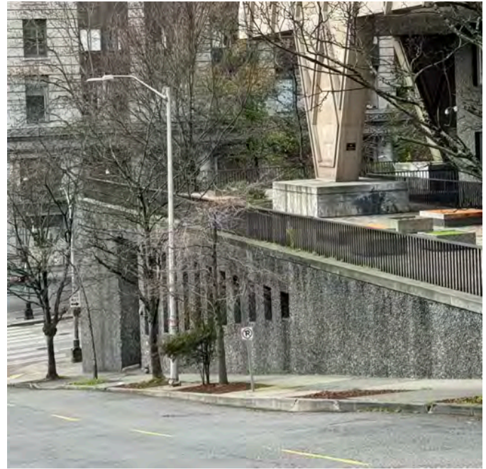
Photograph of Jefferson Street illustrating the steep slope between 4th Avenue and 5th Avenue along the existing King County Administration Building frontage.
