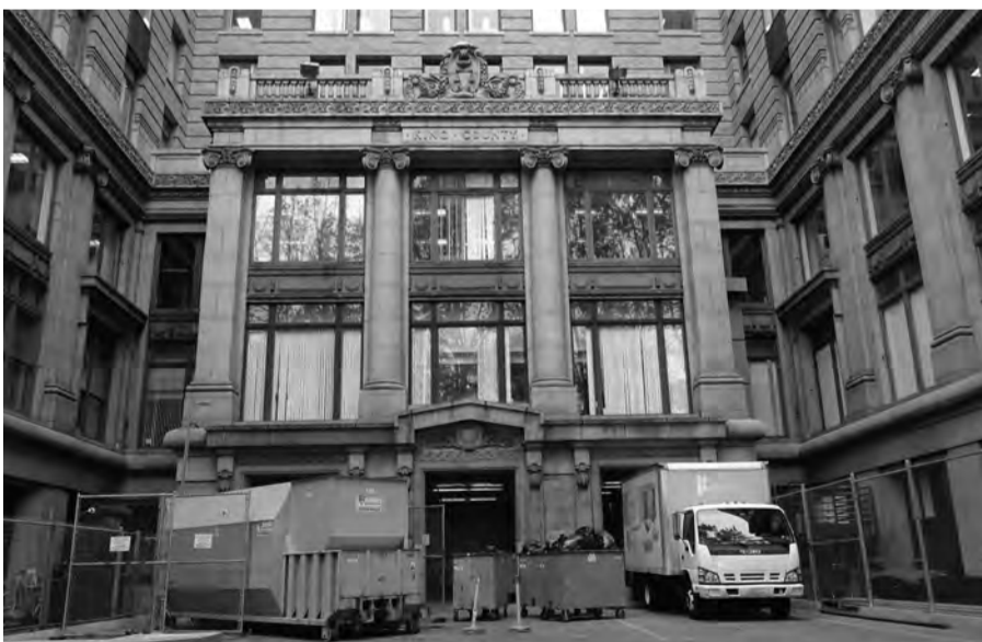
Above: The former main entrance to the King County Courthouse is currently a service entry and loading dock.
