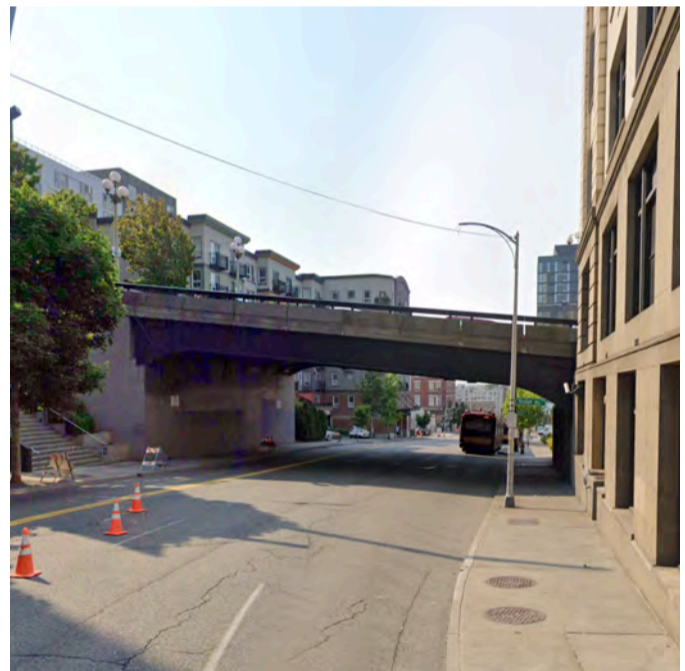
Top: The existing Terrace Street underpass seen from City Hall Park.
