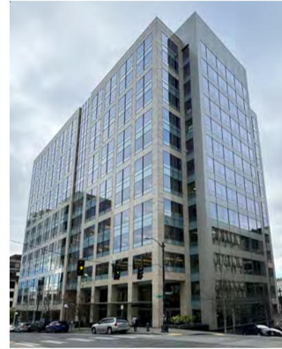
Top: King Street Center, 2023.
