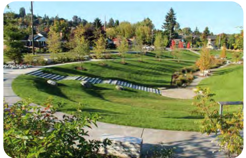
Figure 26. Madison Valley Stormwater Park, Seattle, WA. Stormwater parks provide water quality treatment for stormwater runoff while also adding neighborhood green spaces. Photo source: Seattle Public Utilities, Stormwater Parks & Ponds — Shape Our Water
