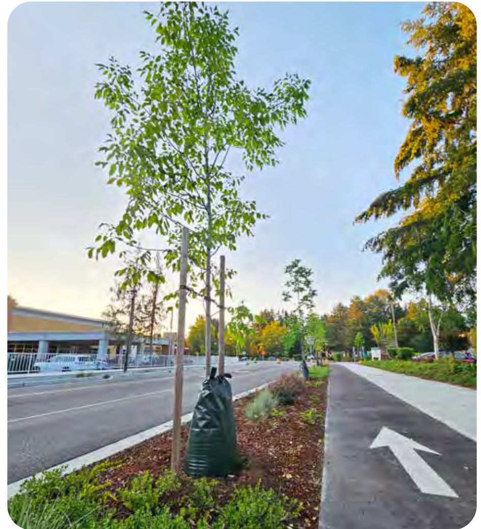
Figure 23. Proper soil volume, staking, mulching, and watering help newly planted trees survive and establish to a healthy mature state. Photo source: King County.
