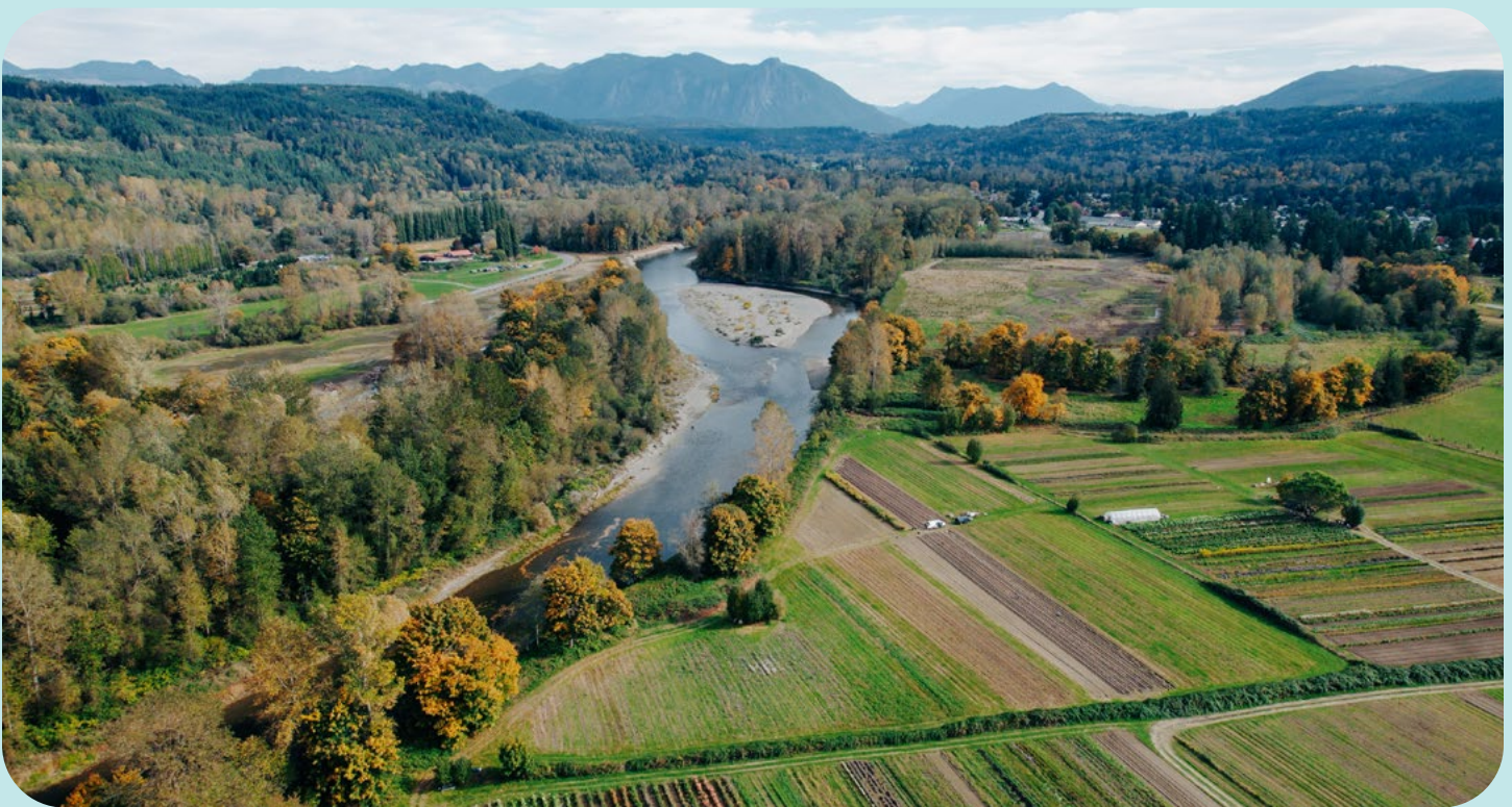
The Fall City Floodplain Restoration Project simultaneously improved habitat and strengthened flood protections for nearby farms, homes, and roads in the Snoqualmie Valley. The project is King County's largest-ever floodplain project.
