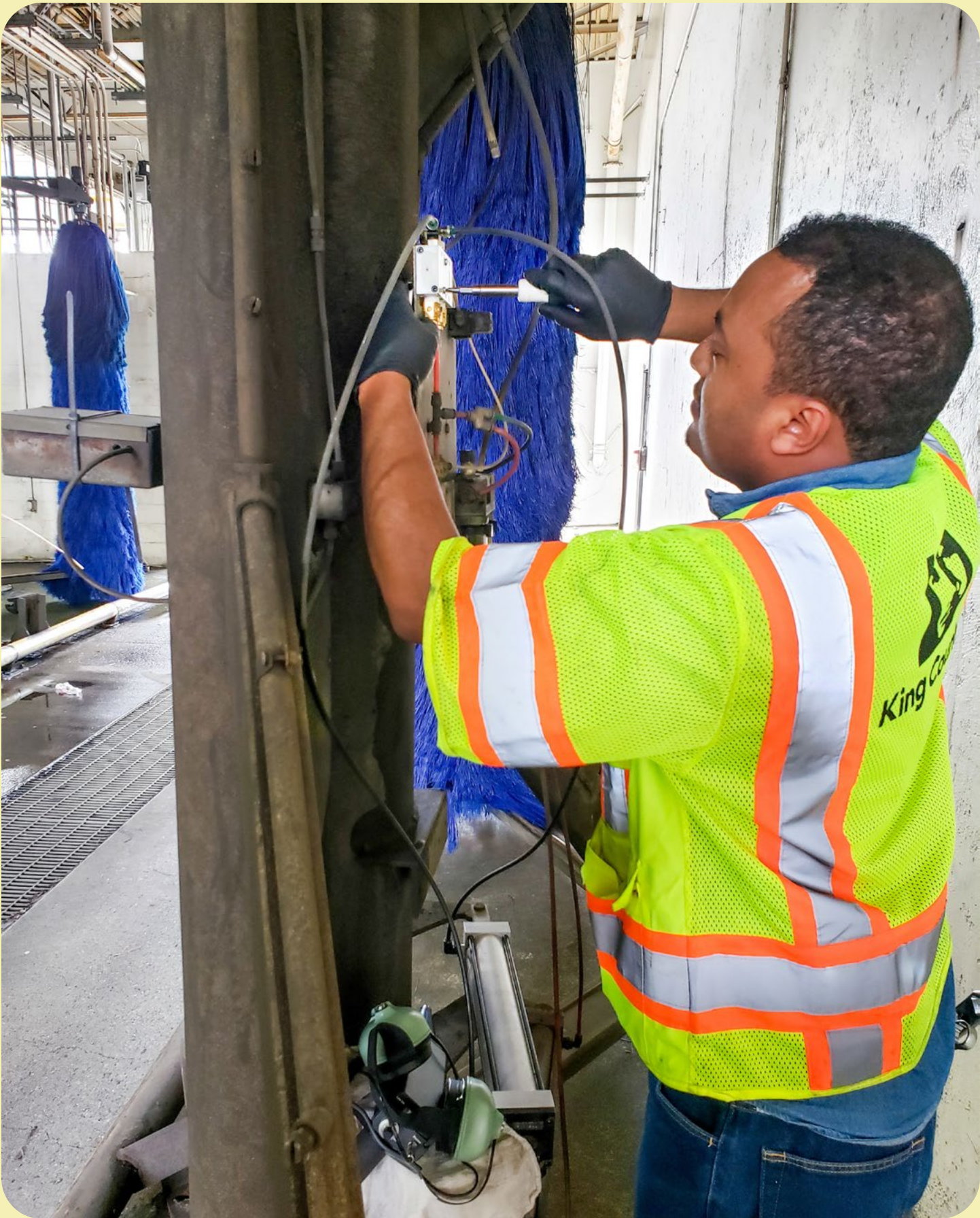
King County Metro Transit employee repairs compressed air leak
