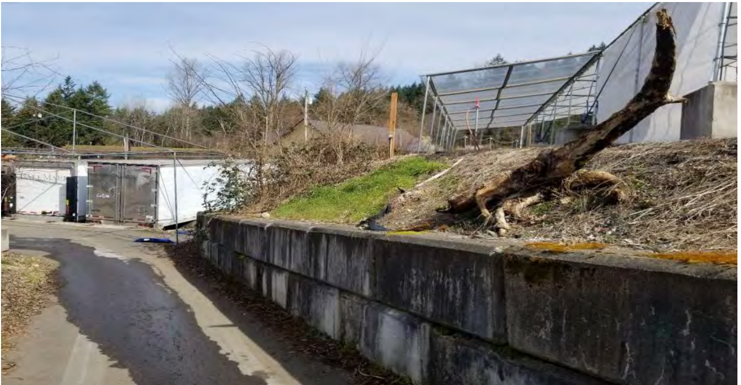
Below: 10' wide asphalt path to loading dock and eco block wall looking north
