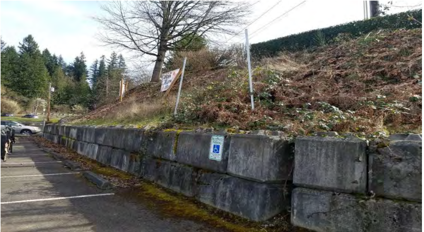
Above: Wall on south side of Parking lot showing Handy-cap stall
