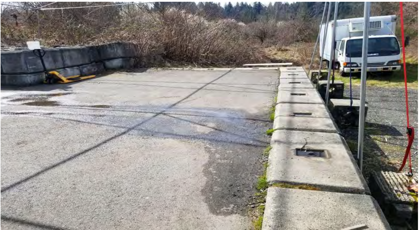
Below: Loading dock looking west
