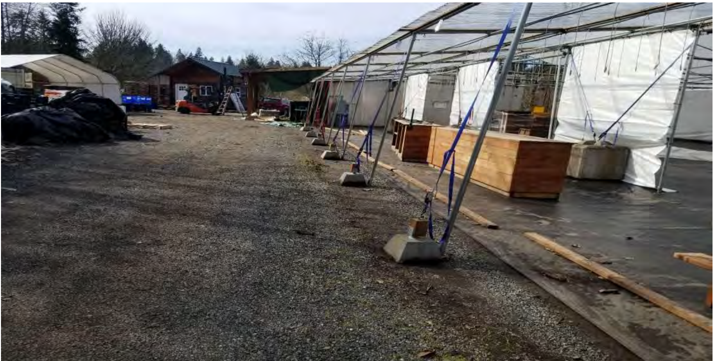
Below: tent die downs and gravel walking / operating path
