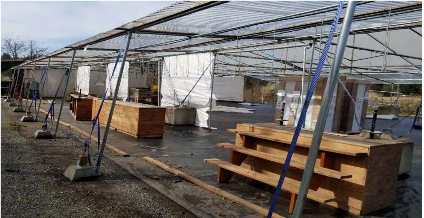
Above: Temp Tent tie downs south side
