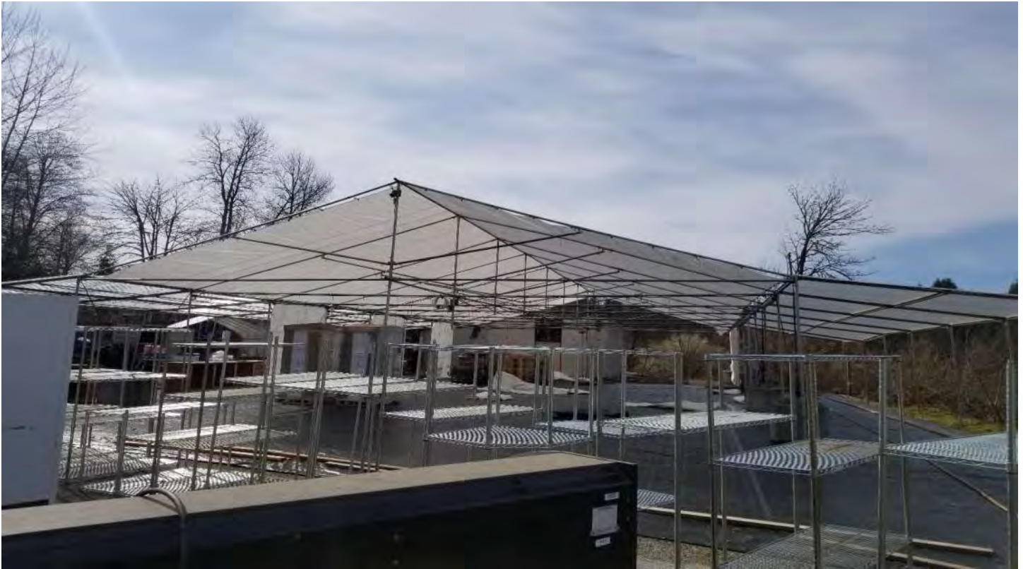
Above: Looking at Temp Tent structure
