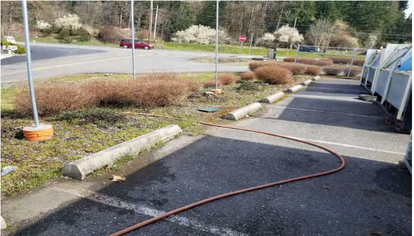
Above: Looking Northeast over northern portion of parking lot and lot drain
