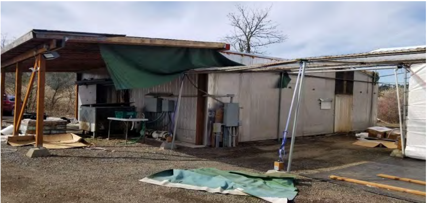
Below: Showing the east side of the Freezer Unit
