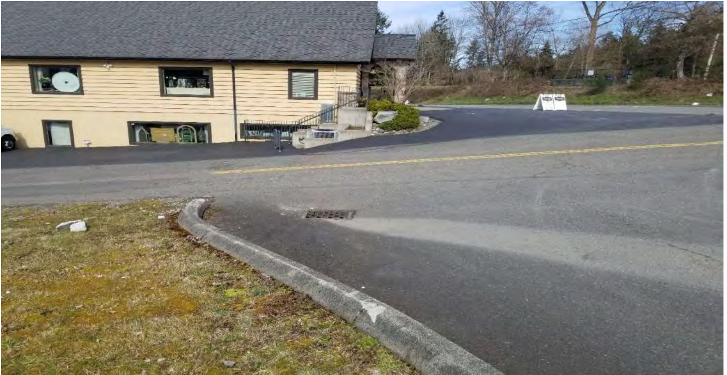
Above: Driveway access showing catch basin looking north
