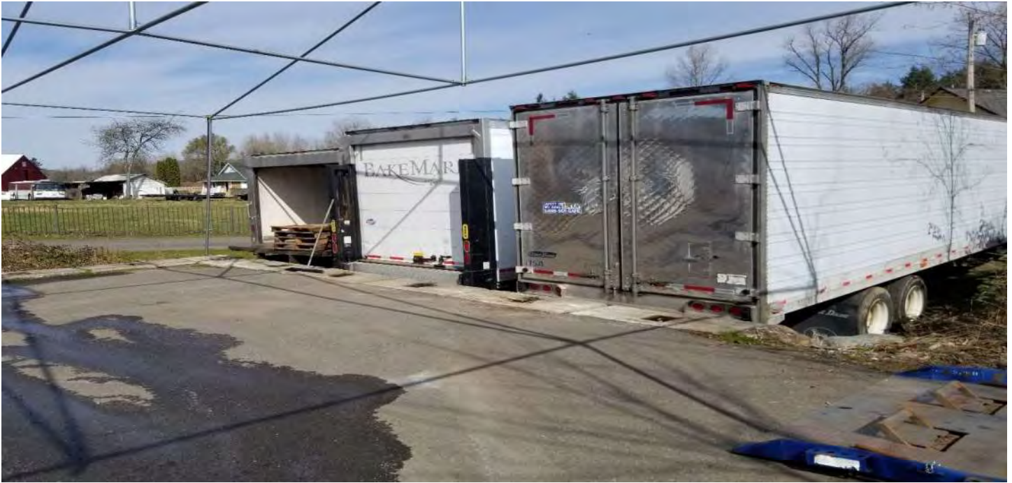
Above: loading dock looking northeast
