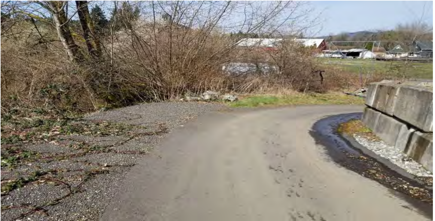
Above: 10' wide asphalt path to loading dock looking north
