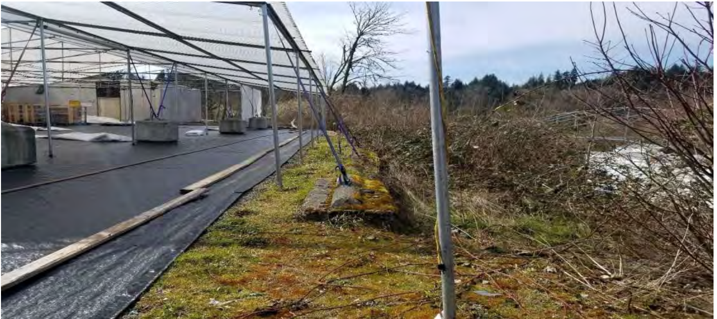
Below: Temp Tent Structure tie-downs north side of tent
