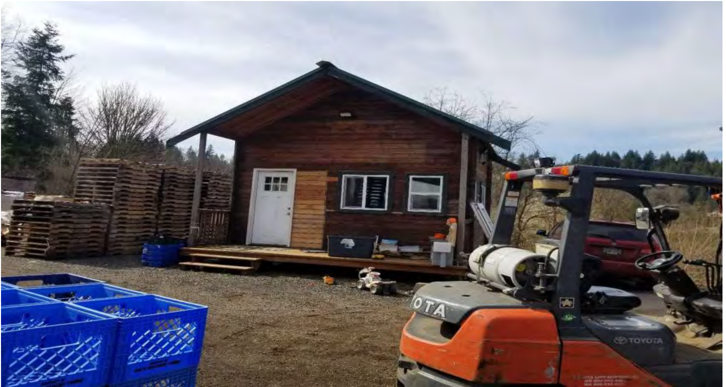
Above: Office Building east side of structure
