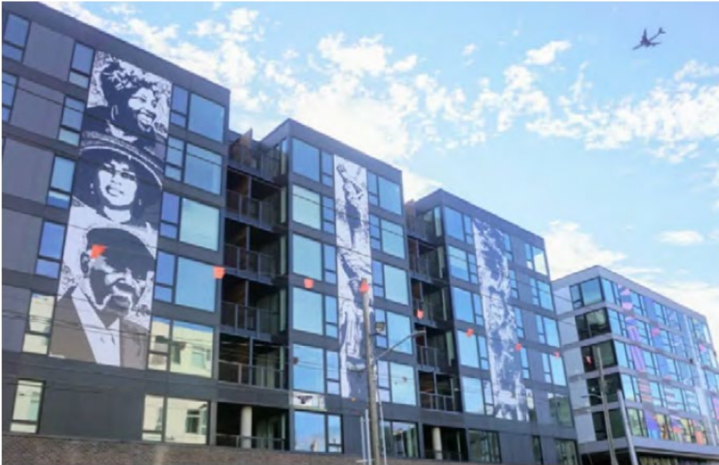
Examples of modulation breaking down building mass. (Midtown Center, by Weinstein A+U and Lake Union Partners)
