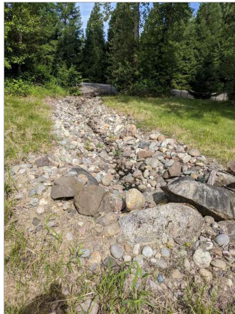
Photo 18. Rock lined ditch facing west towards 240 th Street
