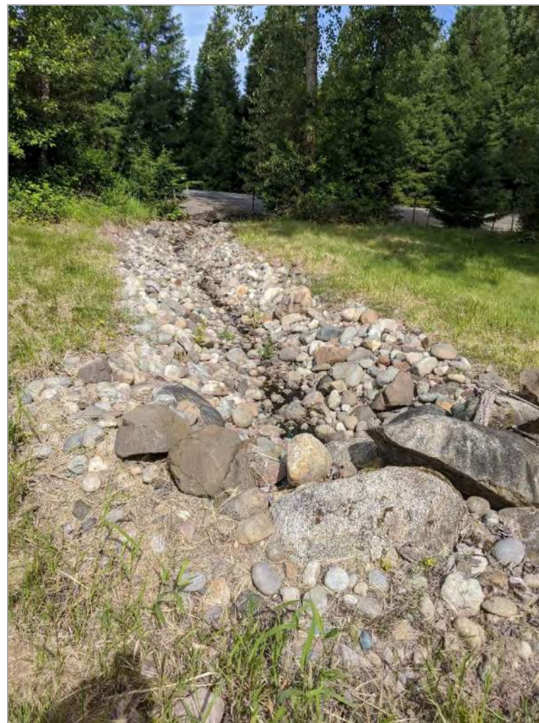
Photo 20. Rock lined ditch facing west towards 240 th Avenue SE
