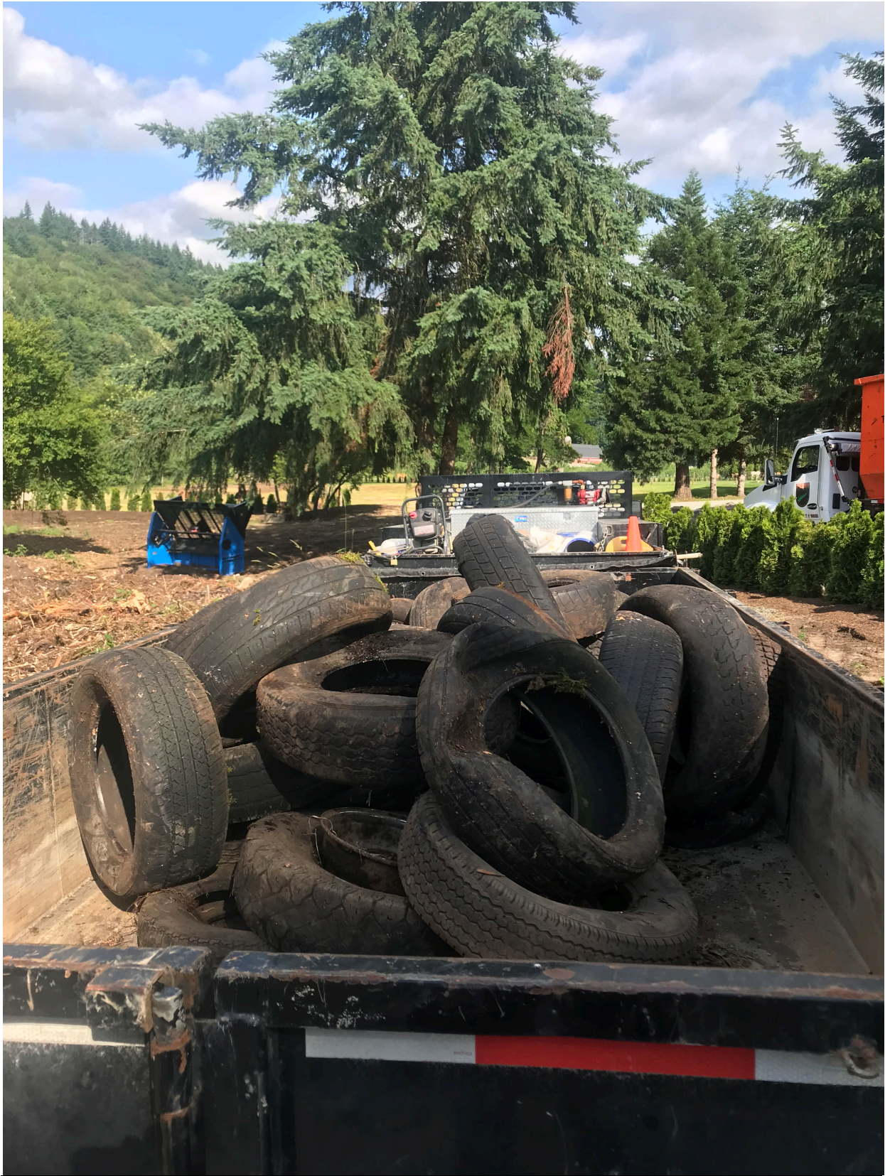
Photo 8 – Removed tires from wetland buffer
