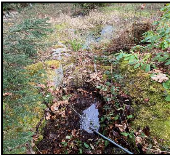
Photo 8 & 9. Photo 8 (left) depicts an elevated concrete basin surrounded by rockery. This basin has collected leaf litter and organic debris but includes pipe at the bottom of the basin that once pumped water to create a fountain. Photo 9 (right) shows a spigot located at the top of a constructed rockery and concrete wall that previously functioned as a waterfall.
