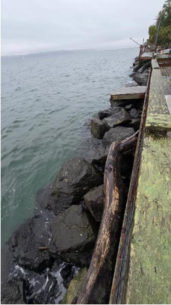
Photo 1: Timber and Rock Bulkhead
