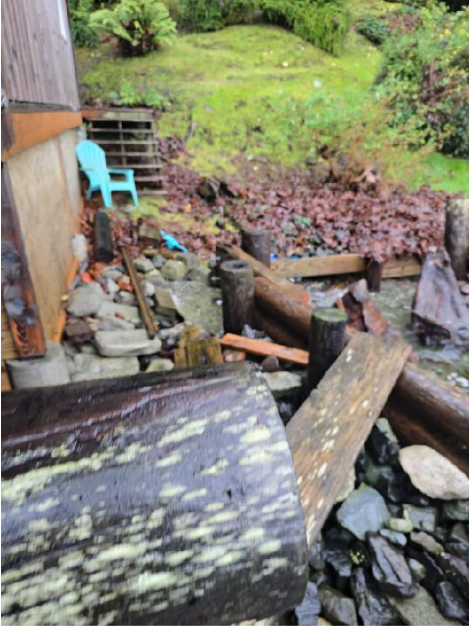
Photo 3: House Located 3 ft From Bulkhead
