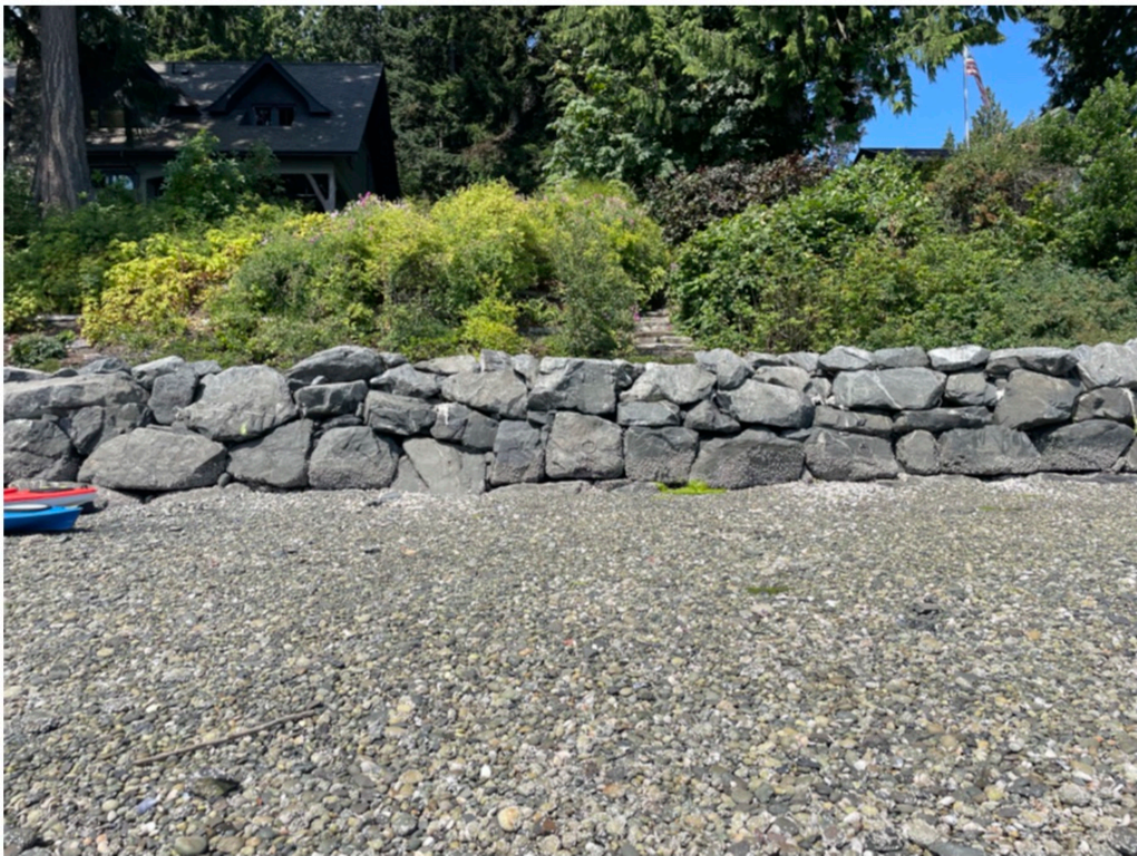
Photo 2 - Shoreline conditions looking shoreward, new pier will extend from rock bulkhead.
