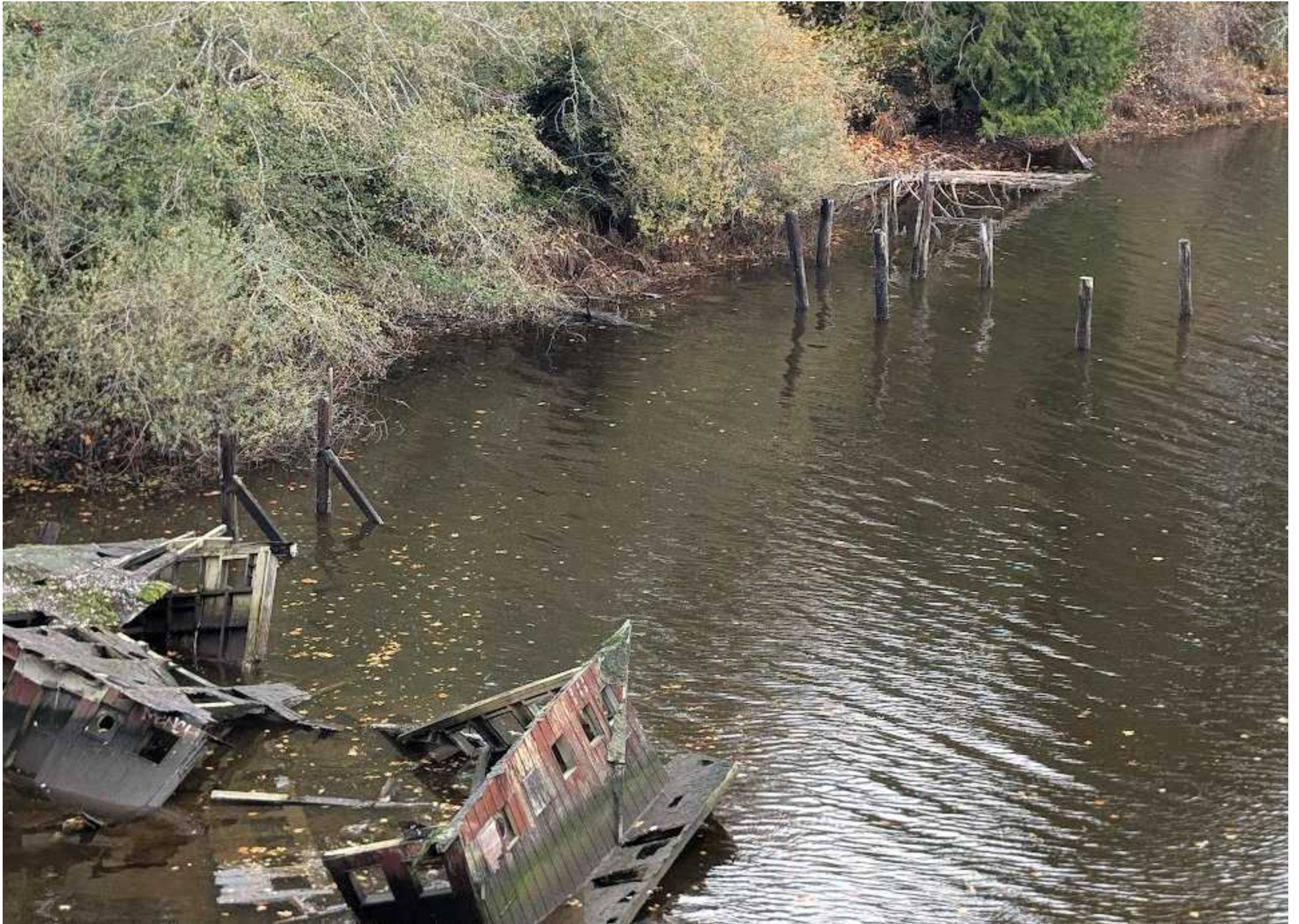
PHOTO OF CREOSOTE PILES TO BE REMOVED (11 TOTAL)
