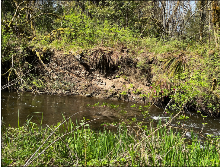
Figure 4. Incised bank/ bank failure on opposite bank.
