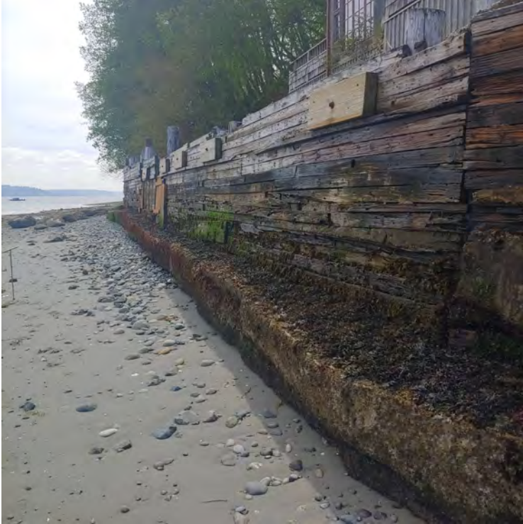
Wood patching and repairs
