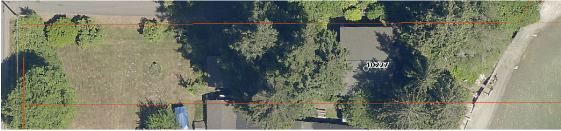
Aerial Photo from King County Website
