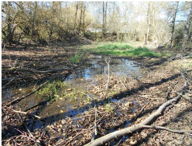
PHOTO 16: LOOKING NORTH ACROSS THE ENGINEERED INFILTRATION POND FROM ITS SOUTHERN BOUNDARY. THE NORTHERN ACCESS ROAD TO THE COMPOST PAD IS LOCATED TO THE NORTH OF THE POND.
