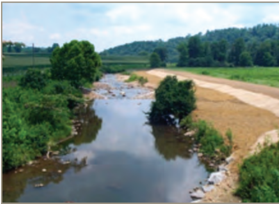
Figure 9.1a Restoration site immediately after construction.
