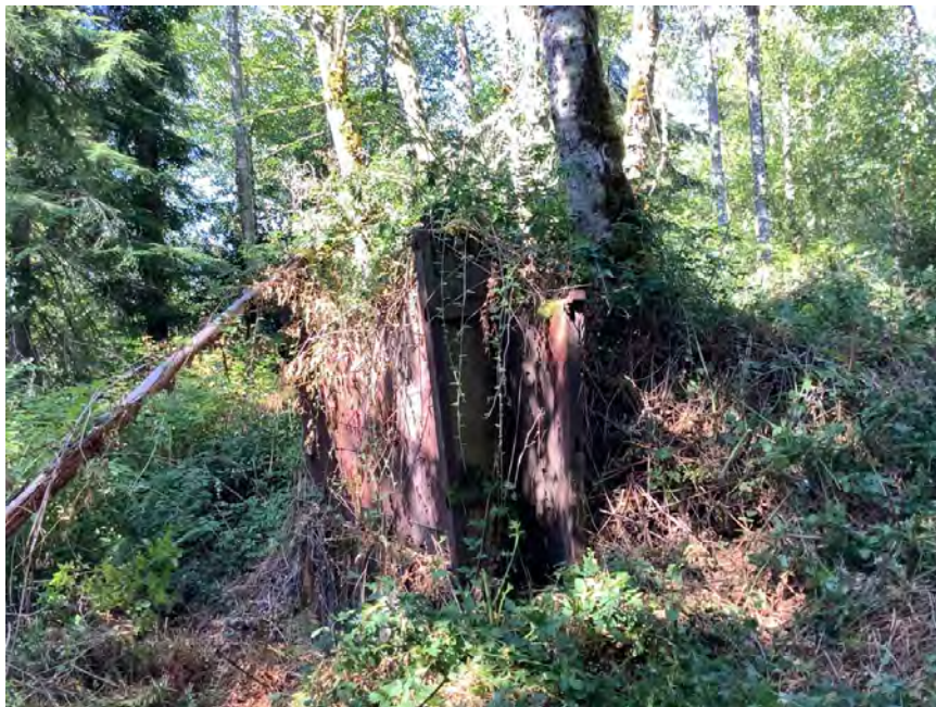
Photograph 4. Former mining infrastructure is visible across the Site.
