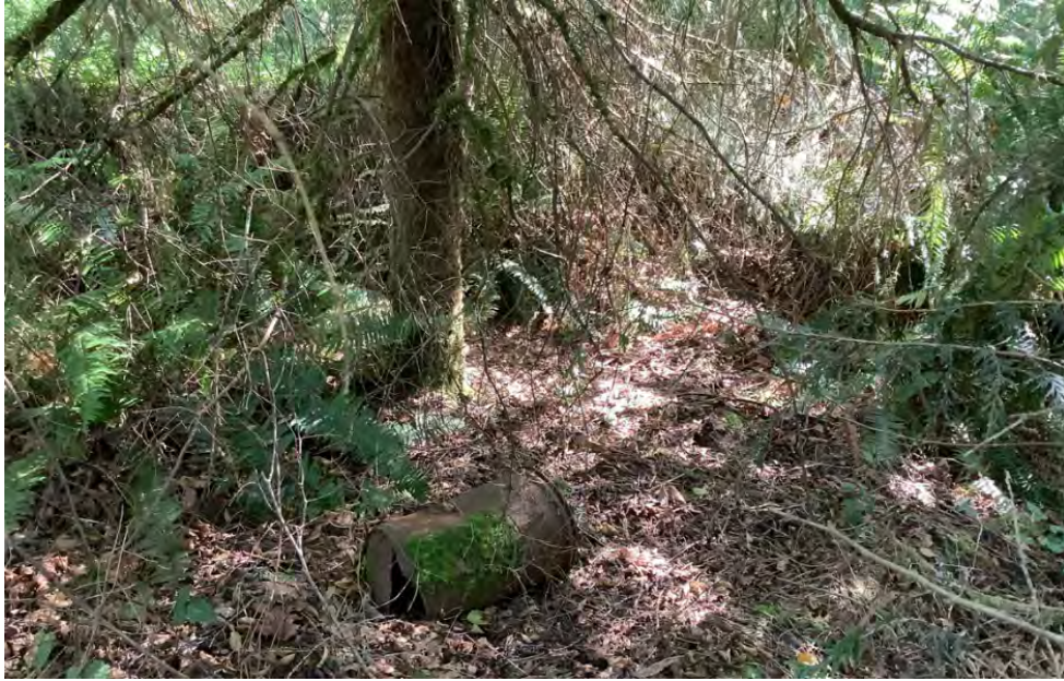
Photograph 5. Several 55-gallon drums and small (< 0.5 gallon) plastic motor oil containers were observed on the south side of the former hearth furnace. The drums were not sealed with lids and appeared to be weathered.
