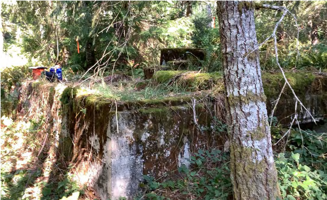
Photograph 3. Foundation and remnants of the former hearth furnace. The furnace was in line with Stockpile 1 and a metal structure (possibly a hopper) to the northwest and Stockpile 4 to the southeast.
