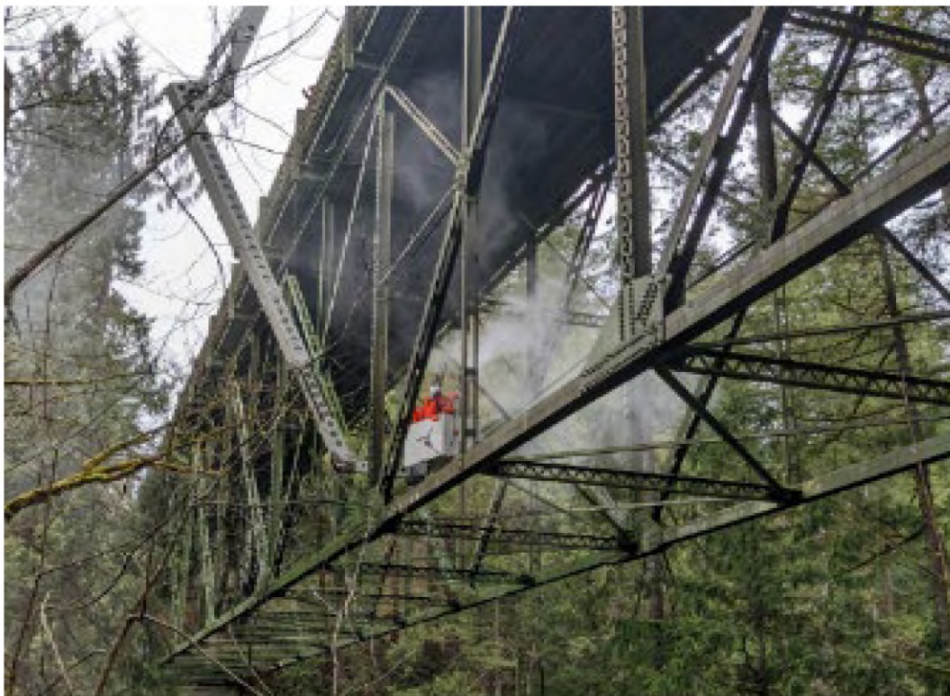
Figure 10: Green River Gorge Bridge No. 3032 - Washing lower truss members in January 2023
