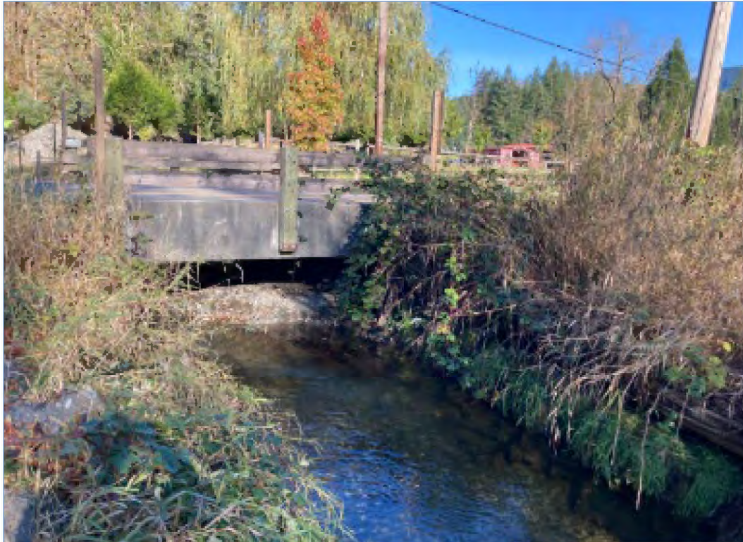
Figure 5: Tate Creek Bridge No. 122N
