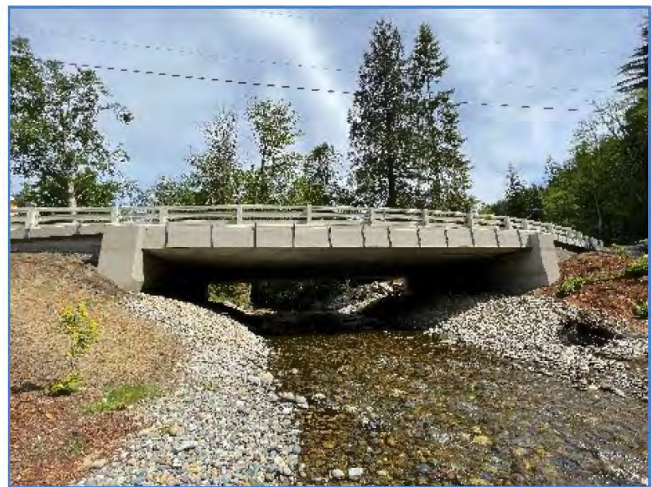
Figure 12: Coal Creek Bridge No. 3035A – New replacement bridge
