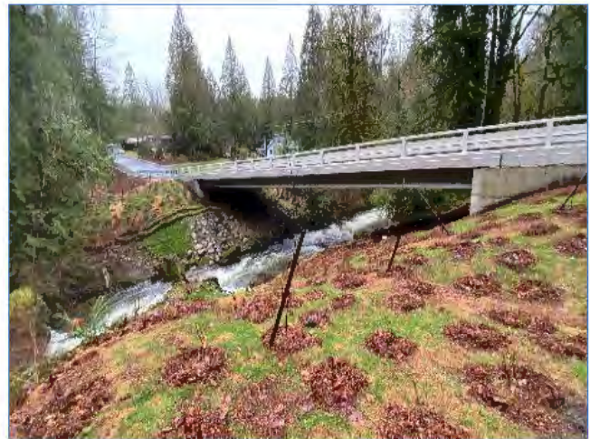
Figure 14: Upper Tokul Creek Bridge No. 271B – New replacement bridge
