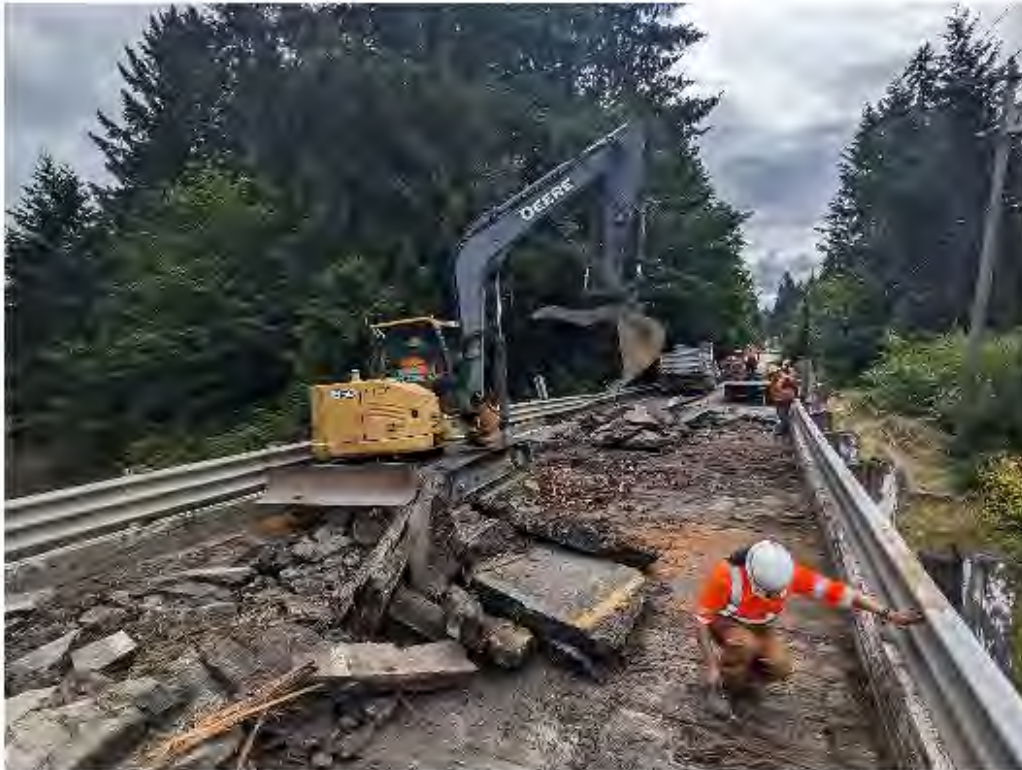
Figure 9: Berrydale No. 3086OX - Removing asphalt overlay to replace timber decking.
