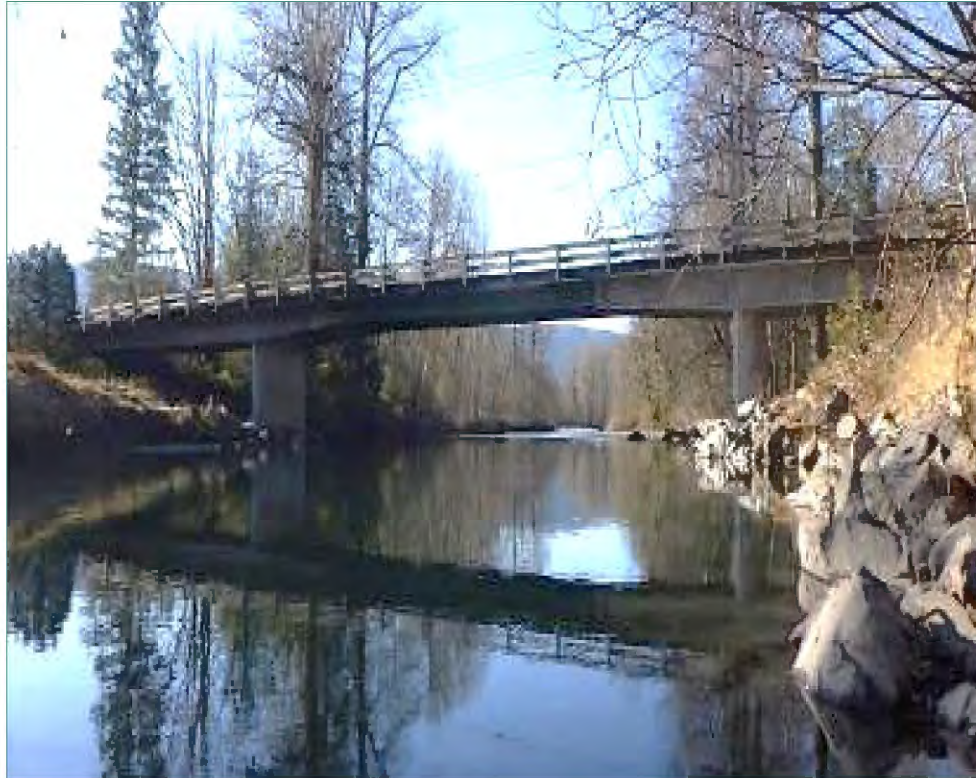
Figure 19: North Fork Bridge No. 122I - Looking south
