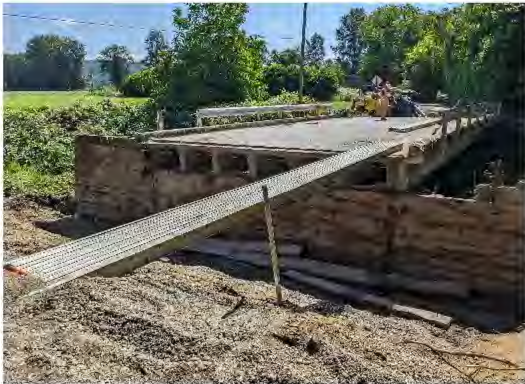
Figure 6: Patterson Creek Bridge No. 228E - Replacing timber abutment and approach roadway.
