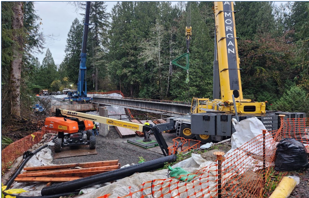
Photo 11: Ames Lake Trestle No. 1320A – Concrete girder launch for new bridge, Nov 2024
