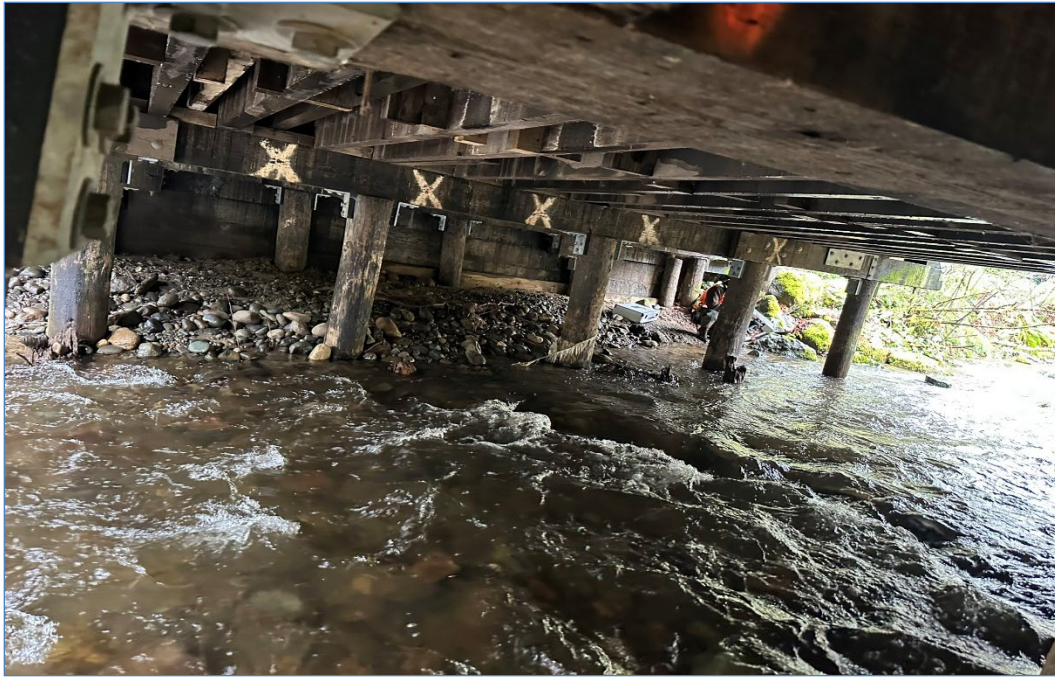
Photo 13: Fifteen Mile Creek Bridge No. 493C - Deteriorating timber superstructure and substructure
