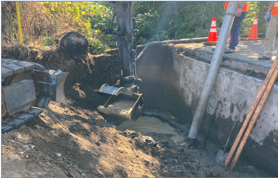
Photo 7: Boise Creek Bridge No. 3051 – exposing scour void
