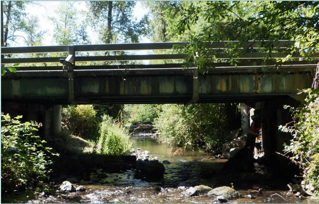
Photo 12: Boise X Connection Bridge No. 3055A - Deteriorating steel girders and timber piles
