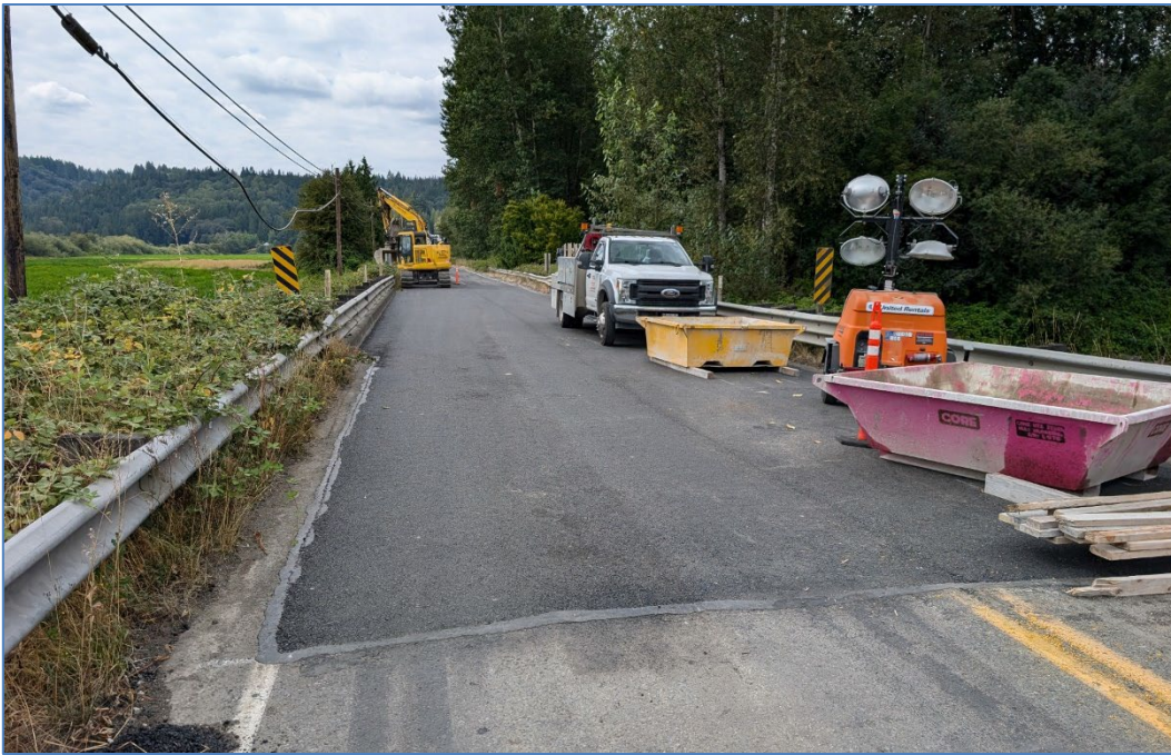
Photo 8: Woodinville – Duvall Bridge No. 1136C – completed overlay
