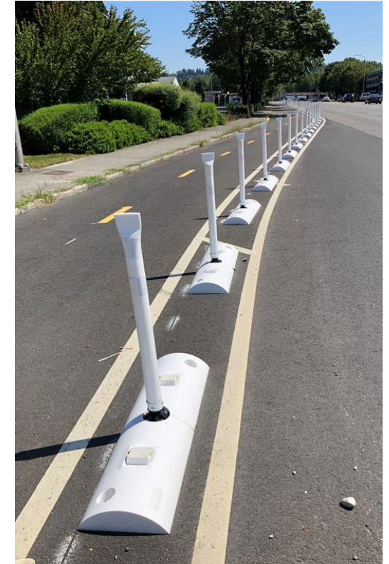
Photo: Tubular marker on curb base
