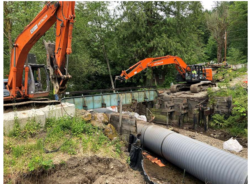
King County Coal Creek Bridge Replacement Project during construction
