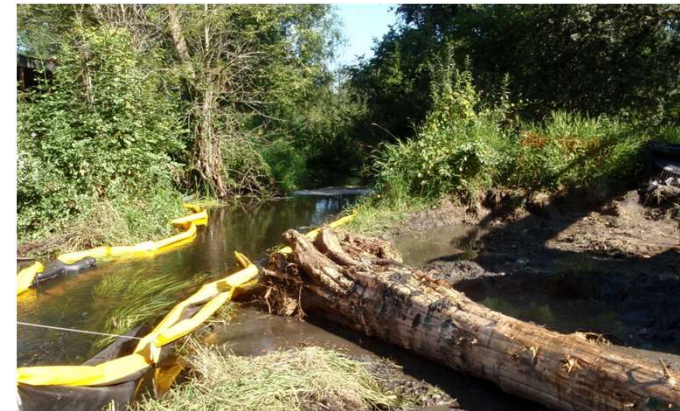
Wood materials as fish habitat at bridge projects near Auburn and Redmond
