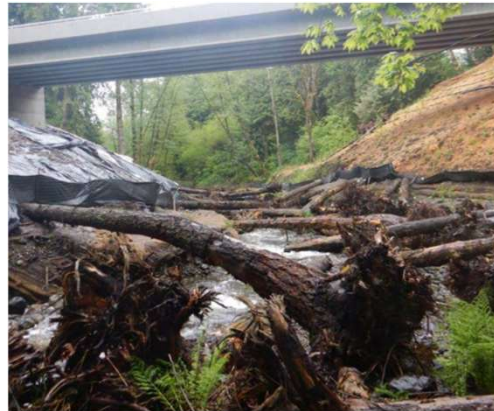
Wood materials as fish habitat at bridge projects near Auburn and Redmond
