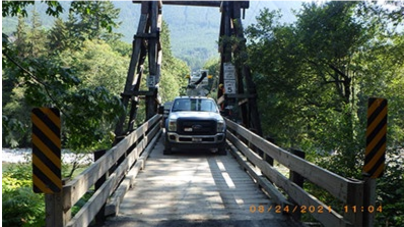
August 24, 2021: Bridge inspectors at work on Baring Bridge.
