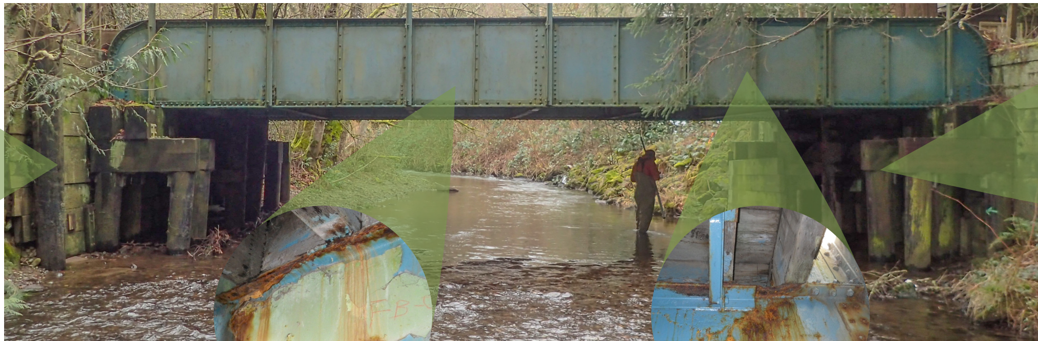
Peeling and flaking paint
