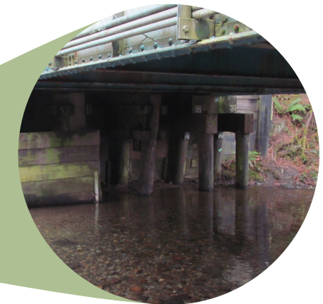
Creosote-treated timber piles in environmentally sensitive creek
