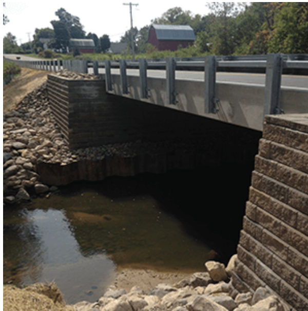
Figure 7-5: Photograph of Sheet Piling Scour Protection
