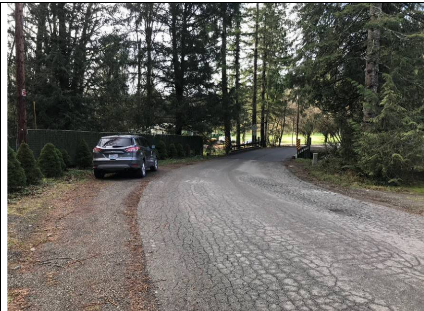
Looking west at the bridge approach/horizontal curve
