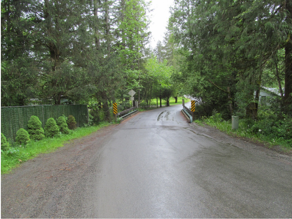
Figure 3-2: Existing Coal Creek Bridge No. 3035A Looking West
