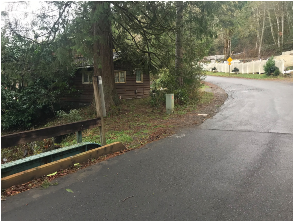
Figure 3-7: Private Residence near Roadway and NE Corner of Existing Coal Creek Bridge No. 3035A
