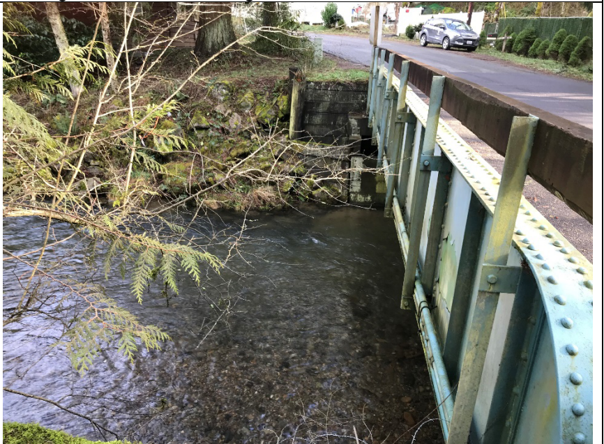
Looking east at the upstream bridge profile
