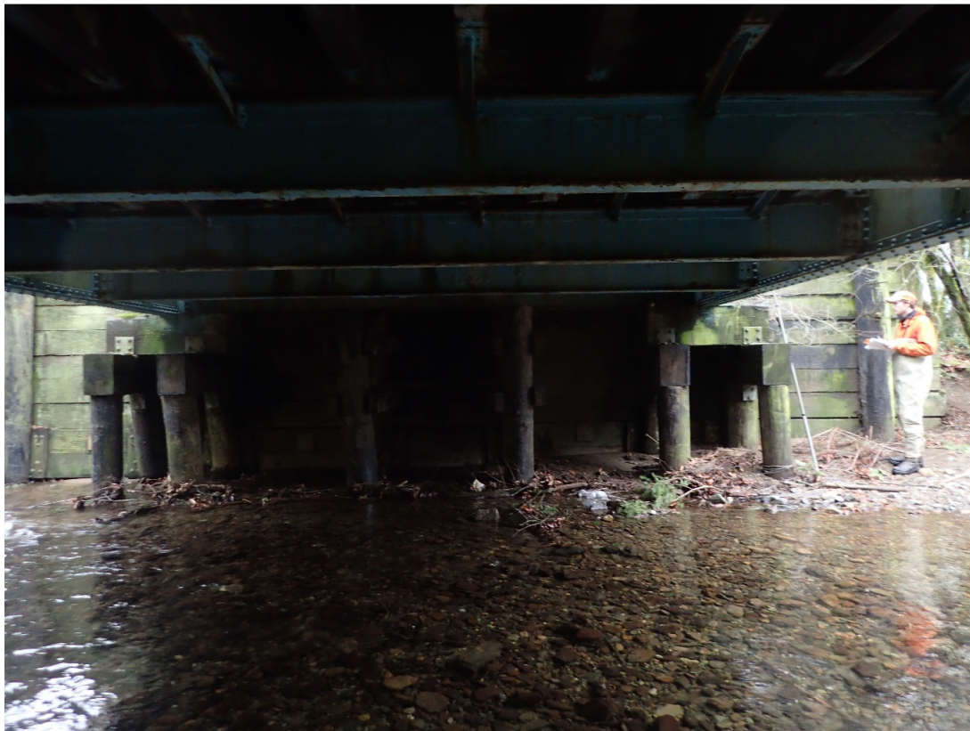
Looking towards RB under bridge (Photo F)
