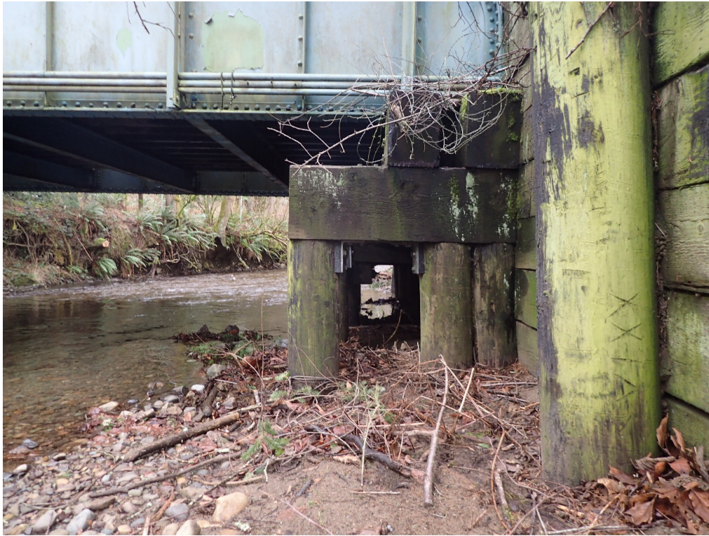
Looking downstream on RB (Photo C)
