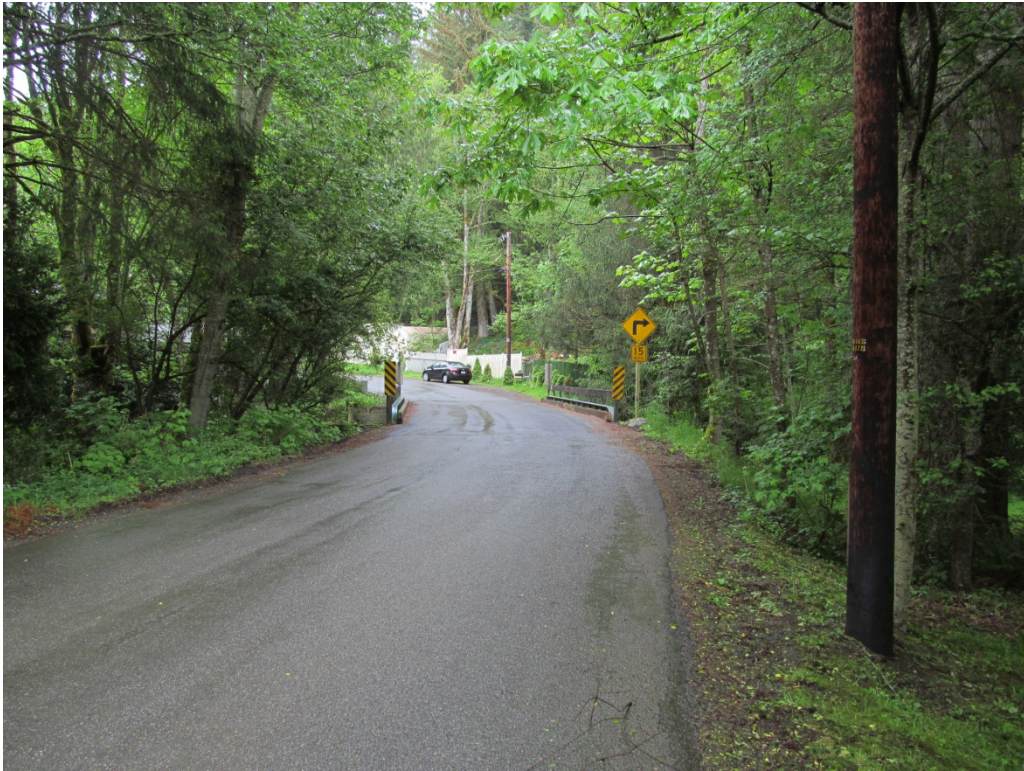
Figure 3-3: Existing Coal Creek Bridge No. 3035A Looking East
