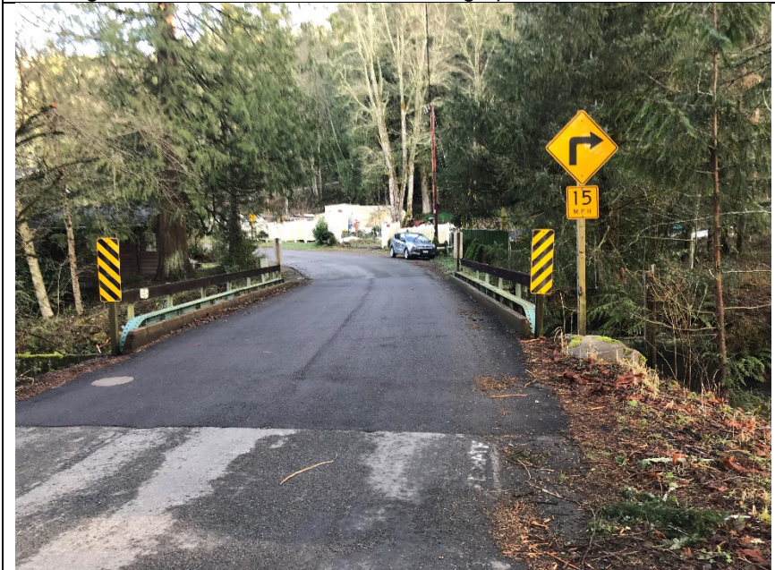
Looking east at the bridge deck
