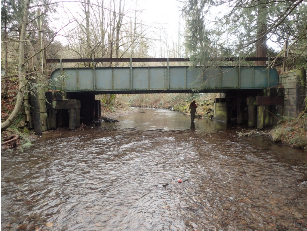
Figure 3-6: Existing Coal Creek Bridge No. 3035A Looking North
