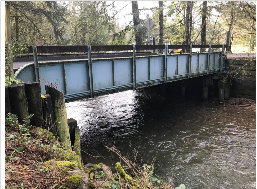
Looking southwest/downstream at the bridge profile
