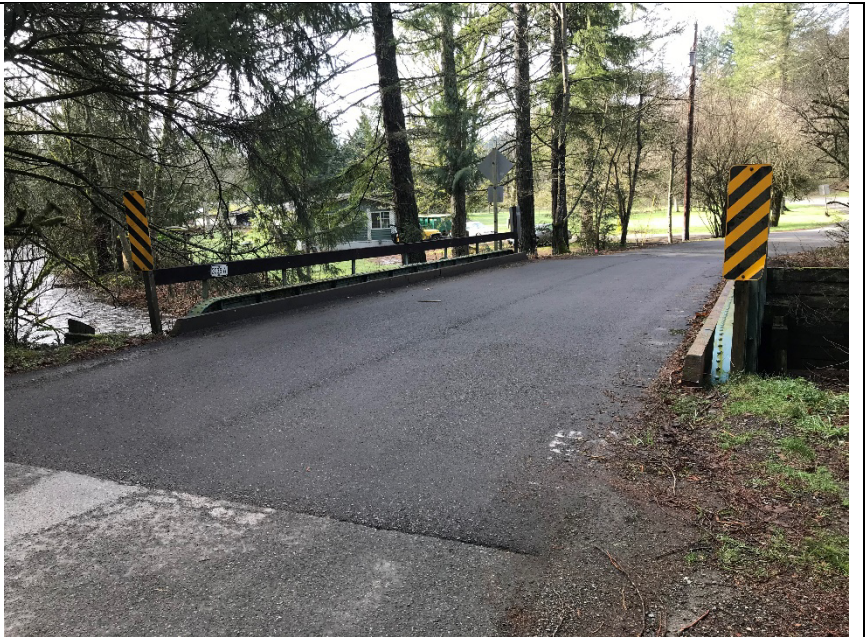
Looking southwest at the bridge deck
