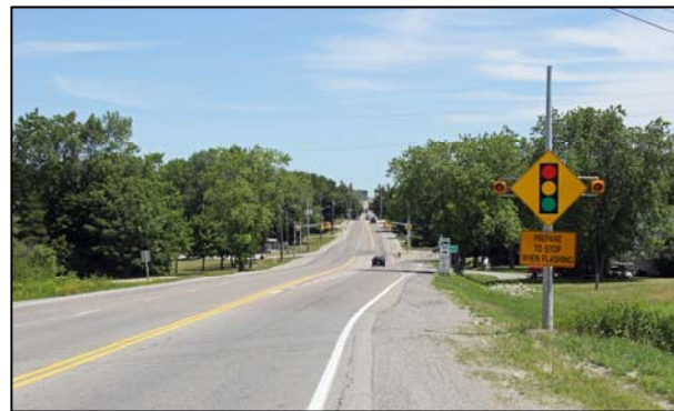
A Prepare to Stop When Flashing sign.
