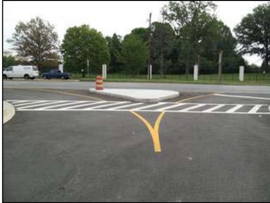
A restricted right-in, right-out example.
