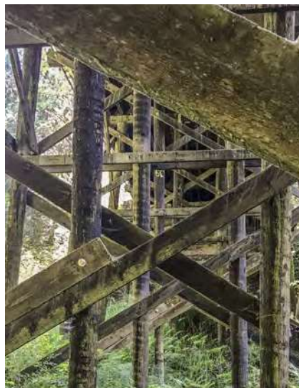
Bridge timber structure is over 100 years old.
