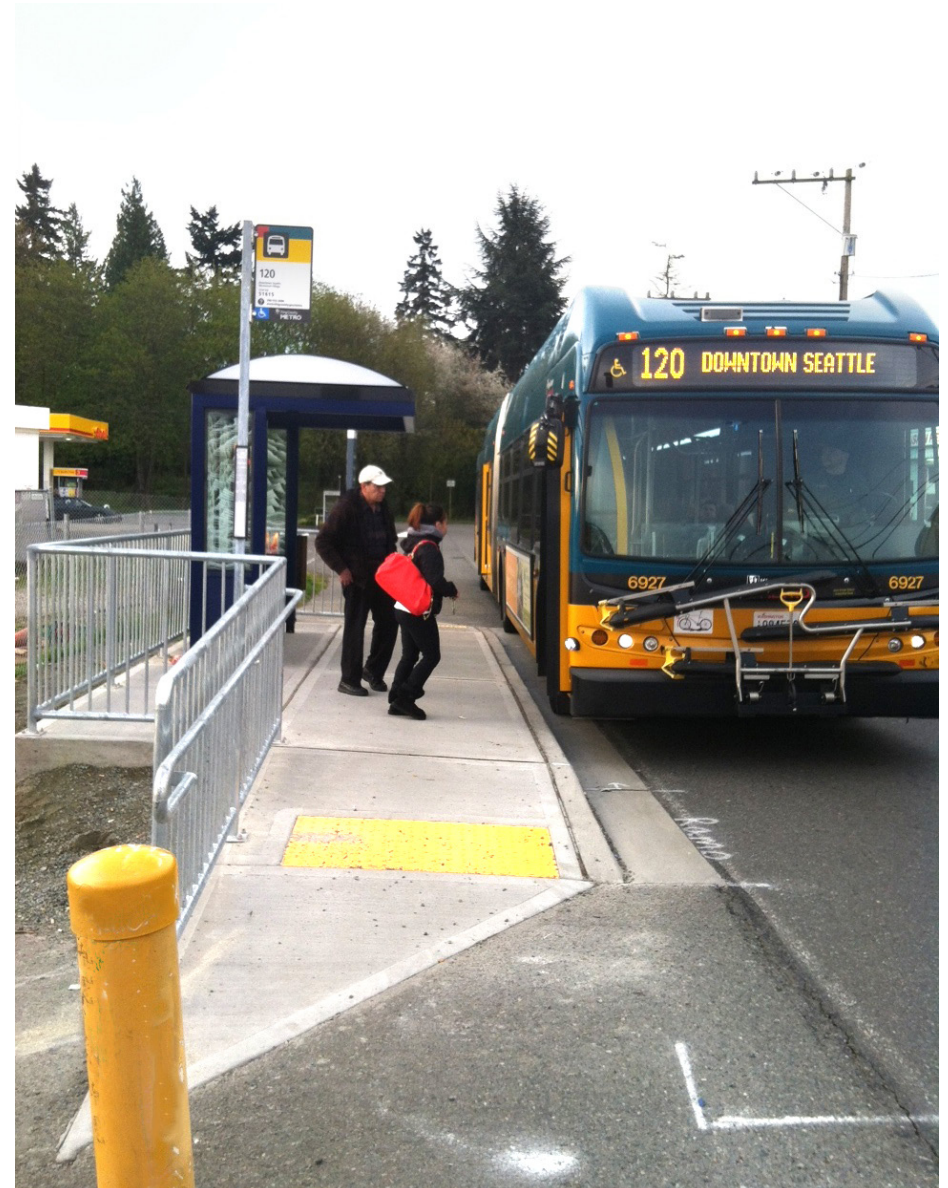
Guardrail at a Raised Landing Pad
