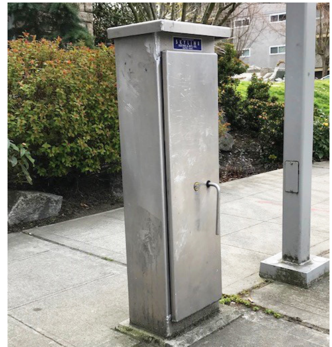
Power Pedestal at a Bus Stop
