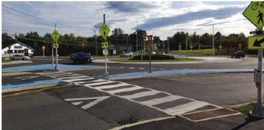
Figure 4: Example of a raised crosswalk at a multilane roundabout (source: NCHRP 1043, Jonathan French). AutoTurn Vertical Clearance Analysis should show minimum 4” clearance for the Metro bus.
