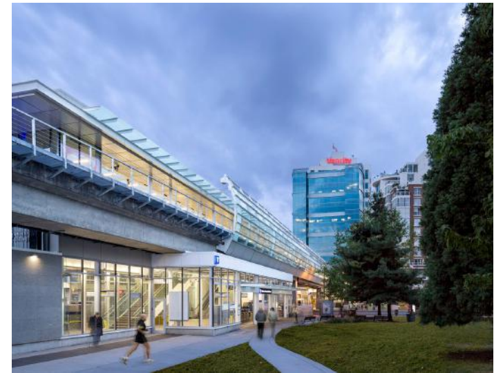
The Main Street - Science World Station was the focus of a recent transit and pedestrian corridor plan in accordance with TransLink's Transit-Oriented Communities policy. (Image courtesy of TransLink)
