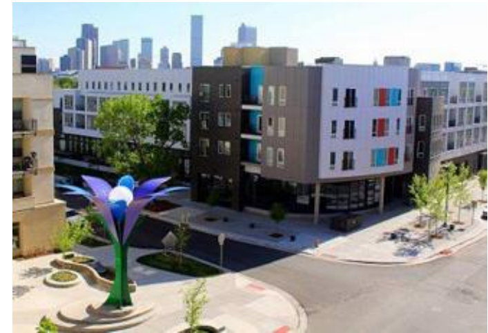
The Mariposa District in Denver is an equitable TOC surrounding the 10th and Osage light rail station. (Image courtesy of Enterprise Community)
