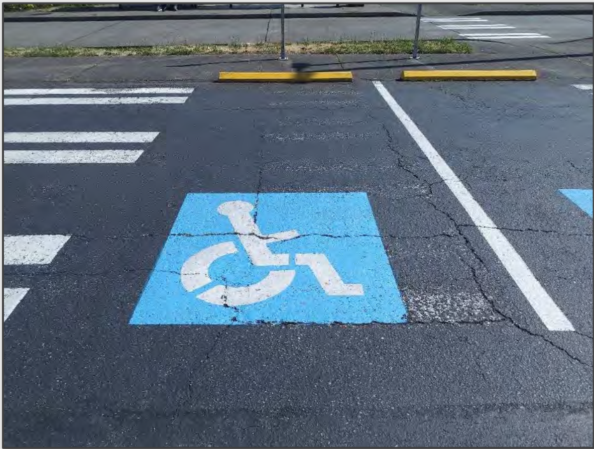
Figure 9: Vertical discontinuities present in accessible parking space
