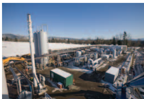
BioEnergy Washington’s renewable energy facility, fueled by landfill methane, at the Cedar Hills Regional Landfill
