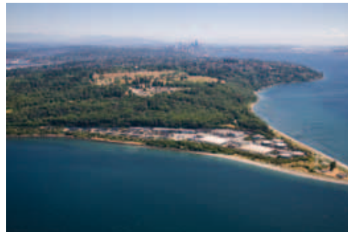
West Point Wastewater Treatment Facility on the edge of the Puget Sound. King County is incorporating the latest science about rising sea levels into planning and operations of the wastewater treatment and conveyance system.
