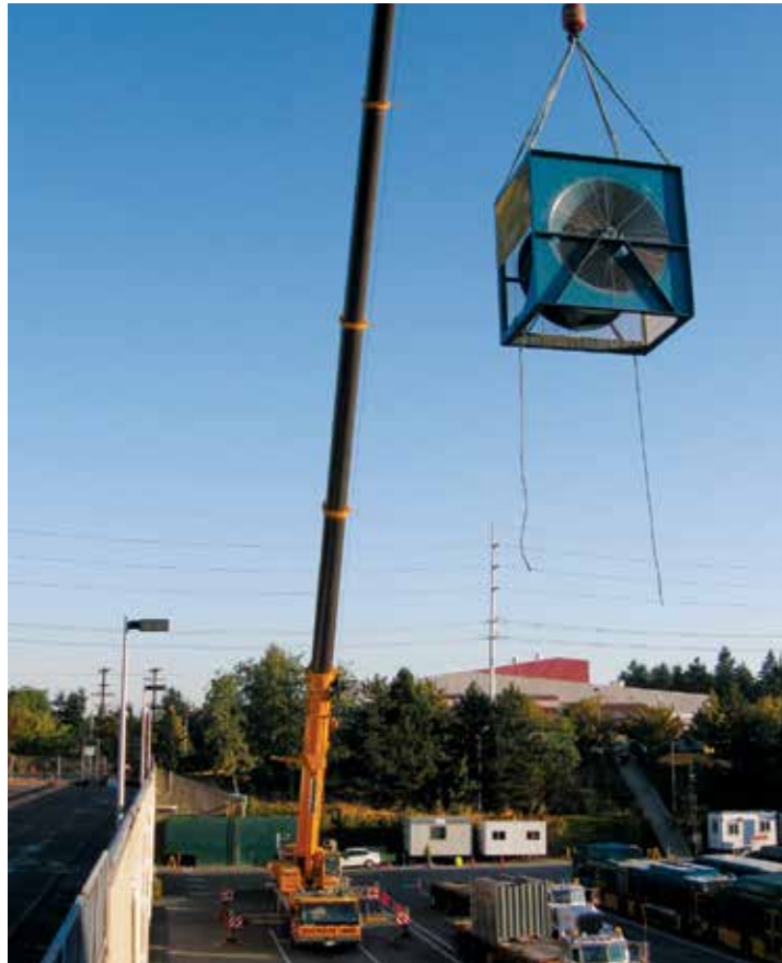
Installing new ventilation fans at the Metro Transit North Base Garage.
