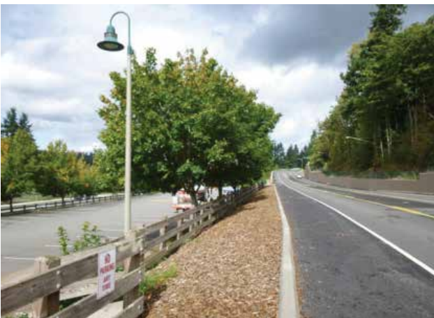
196th Ave. NE at Perrigo Park of the Novelty Hill Road Project showing porous asphalt shoulders
