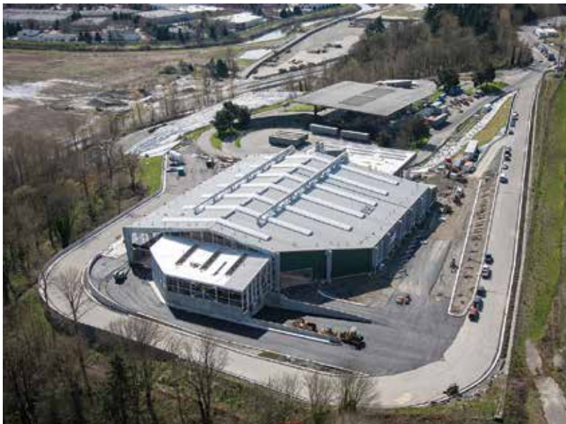
Aerial photo of new Bow Lake Recycling and Transfer Station
